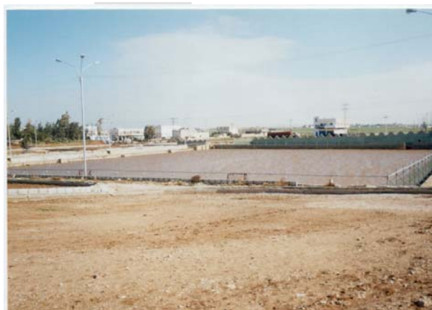
The existing large water pool at Al Jiza
