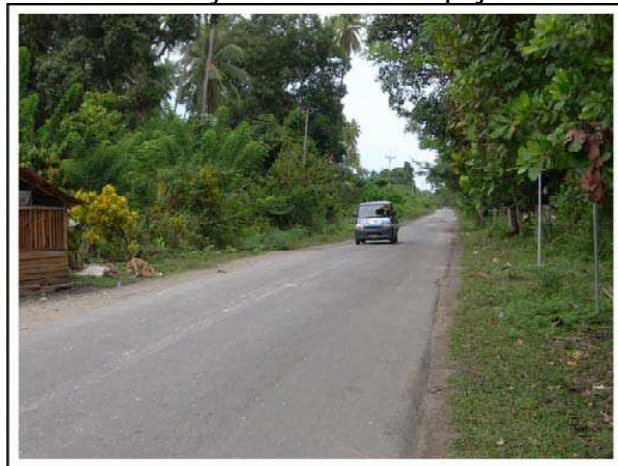
Photo 11. Conditions of State Road that connects Luwuk – Batui
