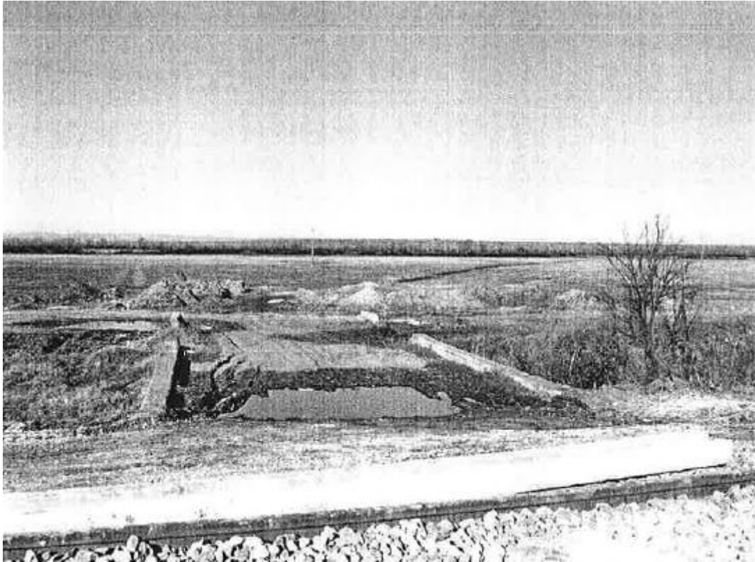
View to the site from south, from the rail track and the station under construction
