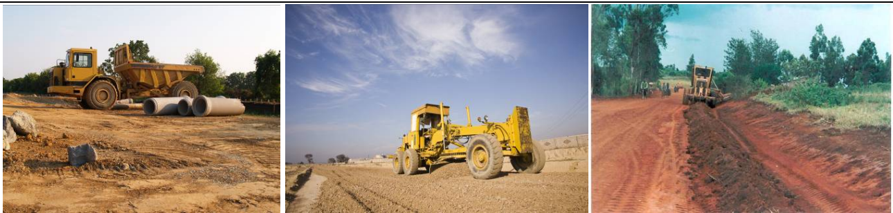
Figure 2.6 Examples of Road Construction
