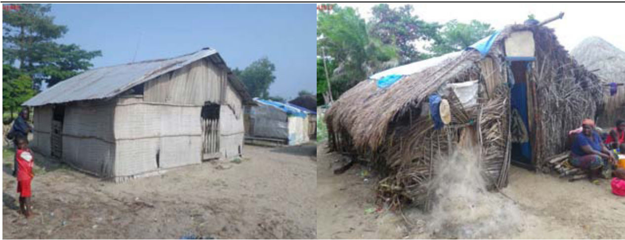
Figure 6.9 Typical Ile Kabak Houses
