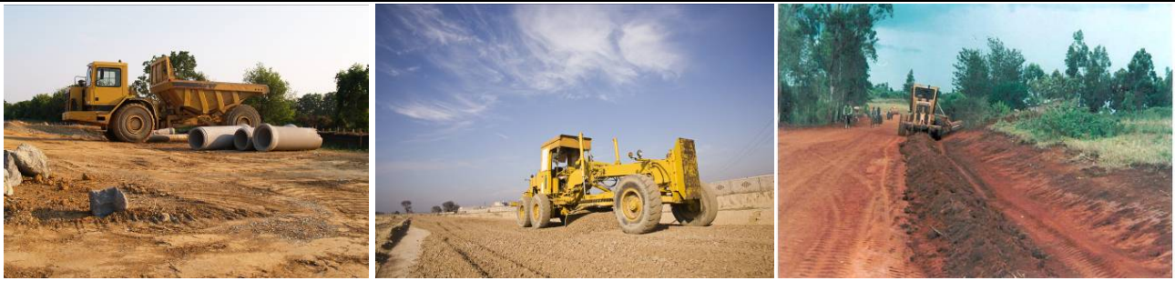
Figure 2.6 Examples of Road Construction
