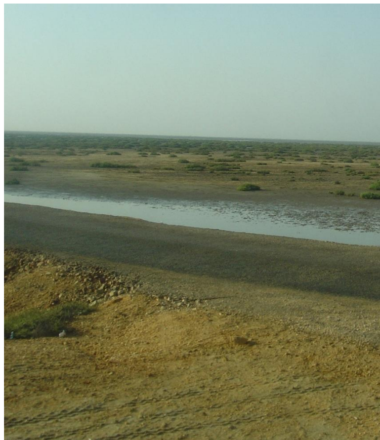
A view of Tanaga wind power project site
