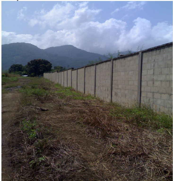
Plate 6: Fence around the Vitafoam property
