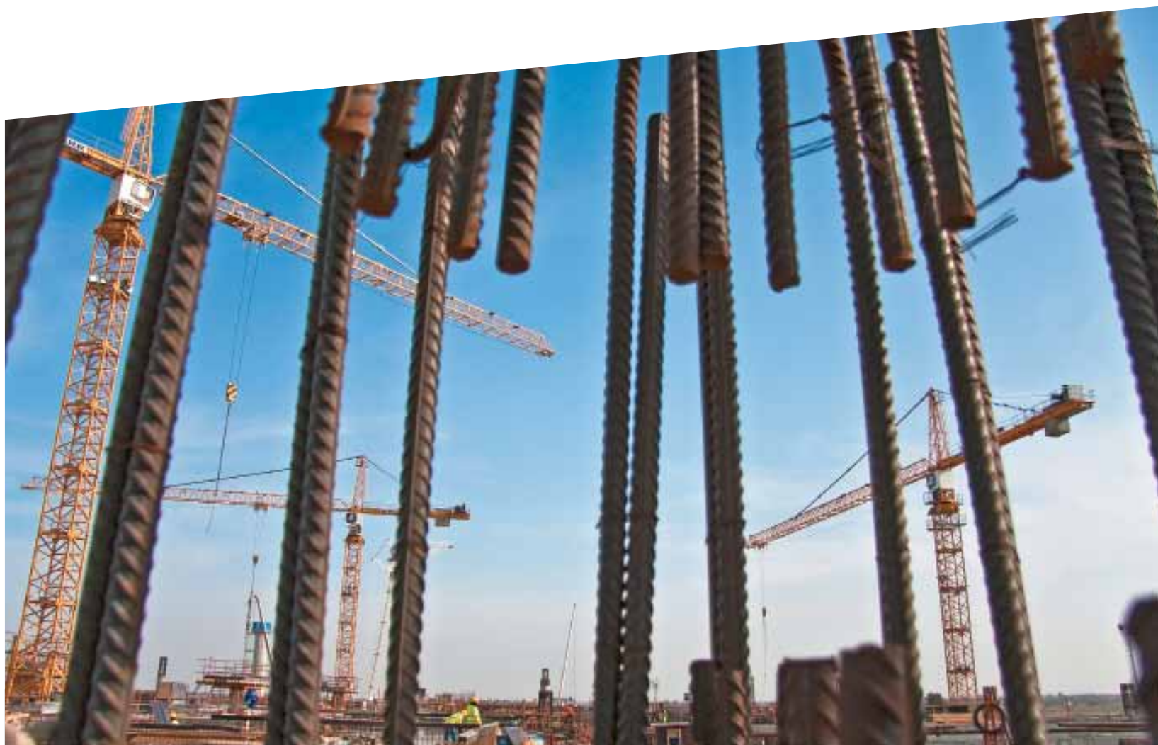
WORKS AT TRIPOLI AIRPORT IN LIBYA
