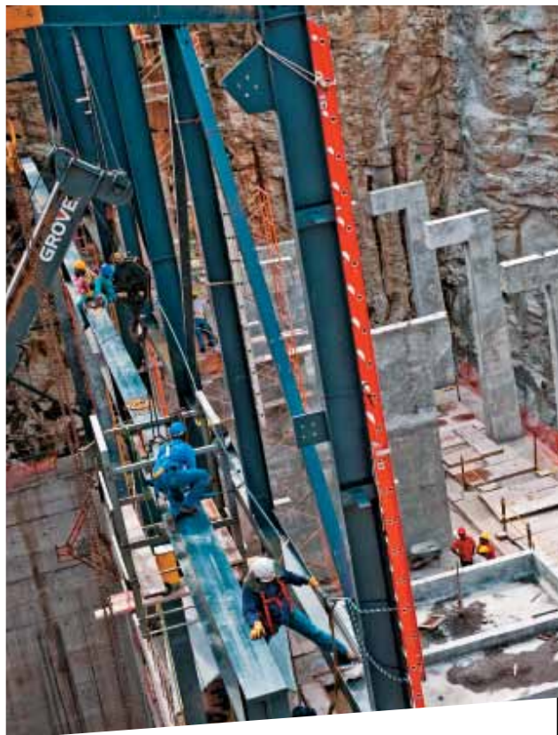
CONSTRUCTION OF THE MARES HYDROPOWER PLANT IN PANAMA
