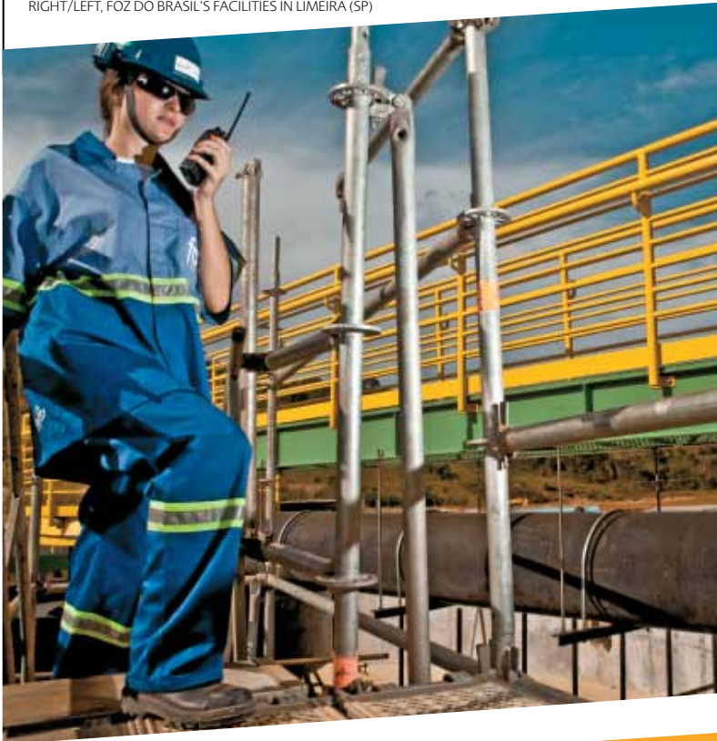
MEMBER OF FOZ DO BRASIL AT THE CONSTRUCTION SITE FOR THE VALLOUREC & SUMITOMO TUBOS DO BRASIL MILL'S UTILITIES PLANT IN JECEABA (MG); RIGHT/LEFT, FOZ DO BRASIL'S FACILITIES IN LIMEIRA (SP)
