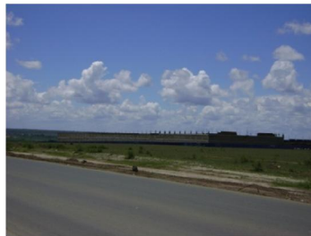
Figure 6: Factory and warehouse for Tile and Carpet Centre
