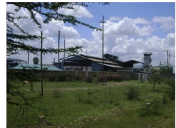
Figure 5: Athi river steel rolling plant
