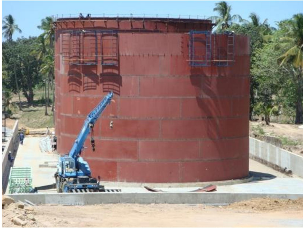
Figure 5-7: Image of typical aboveground HFO storage tanks under construction
