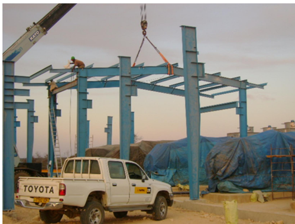
Figure 5-10: Typical image of power house under construction
