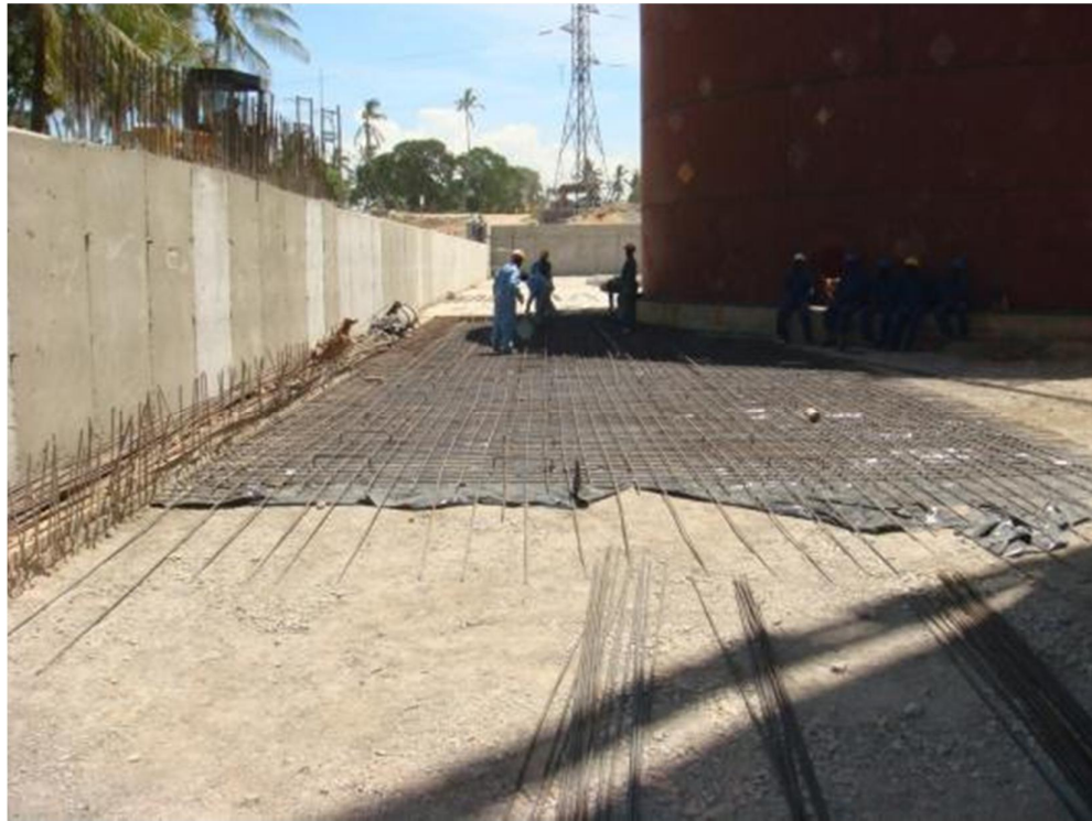
Figure 5-6: Image of a bulk liquids storage tank farm under construction
