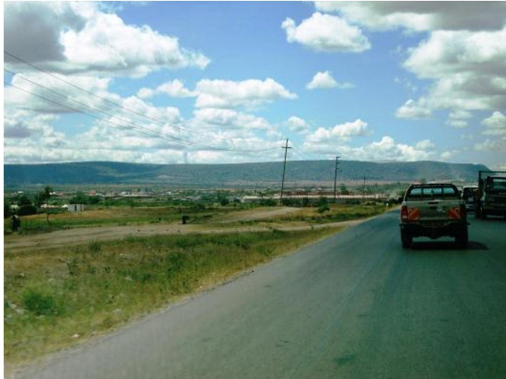
Figure 1-8: Image showing existing 66KV line feeding the ARSP and NCC
