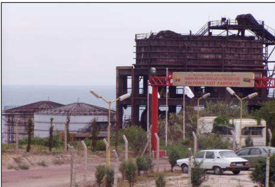
Figure 13 Photo from the ETI Sulphuric Acid Factory
