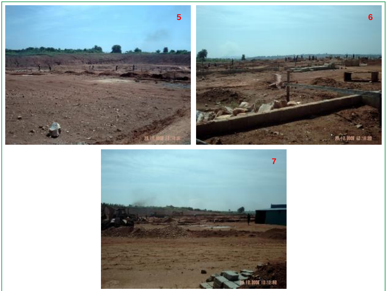
Figure 5: Phase 2 construction activities
