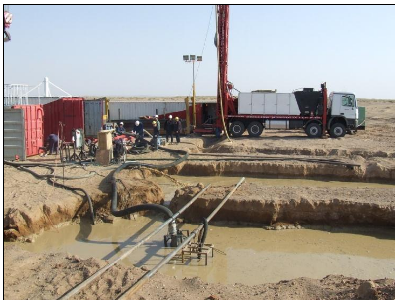
Figure 5.13: Drilling Rig and Infrastructure including mud pits
