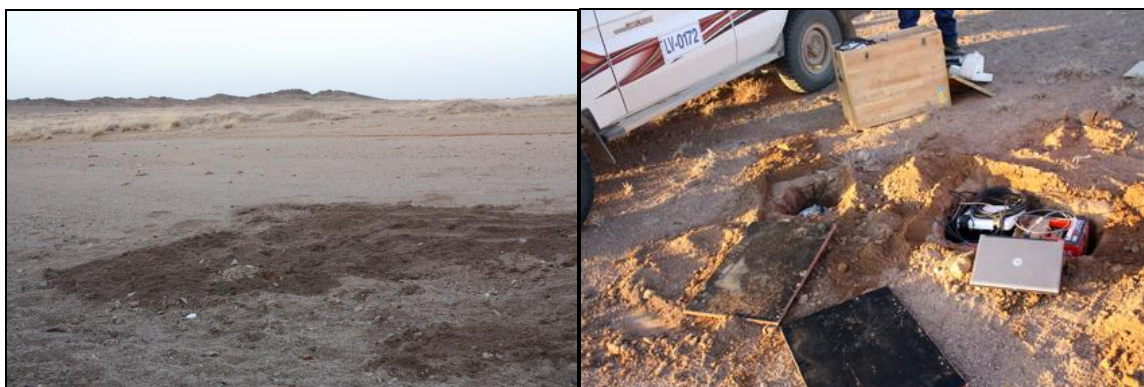
Figure 4.18: Sample Field Installation
