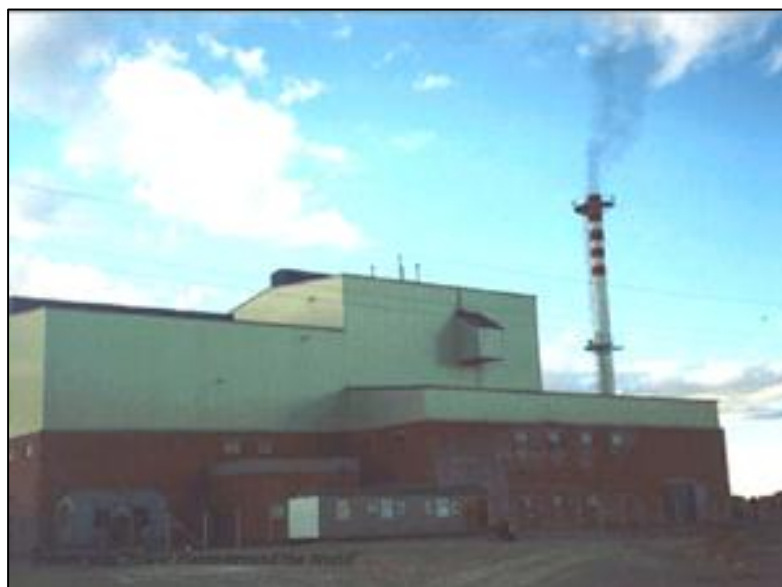
Figure 11.6: Dalanzadgad Power Plant
