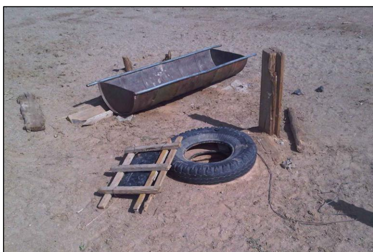
Figure 11.8: Typical Shallow Hand Dug Herder Well
