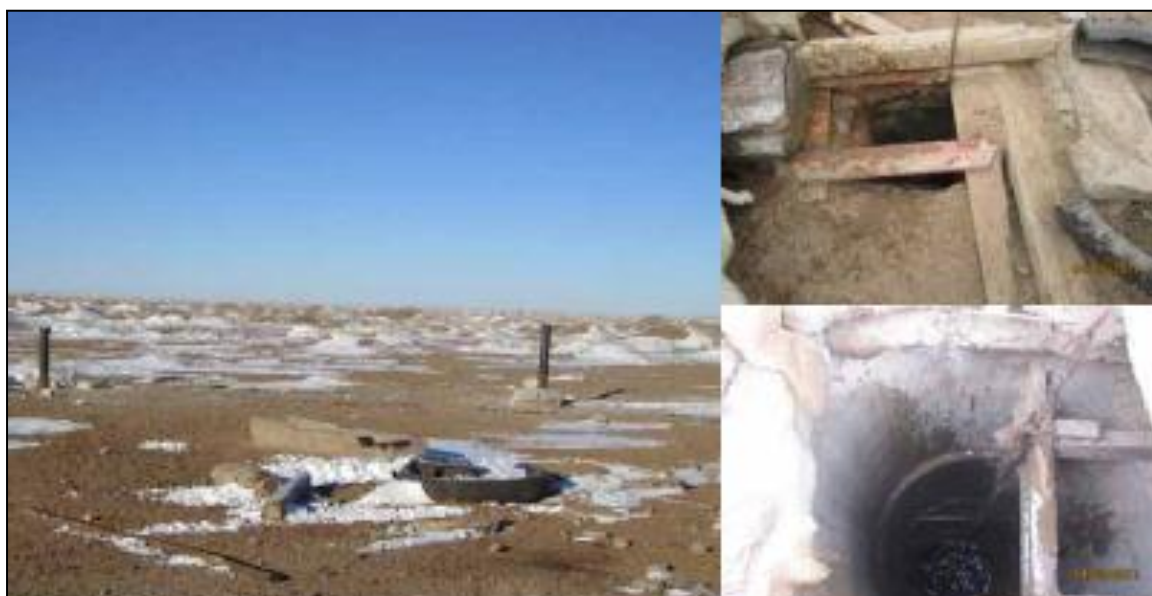
Figure 10.10: Typical Shallow Hand-Dug Herder Well
