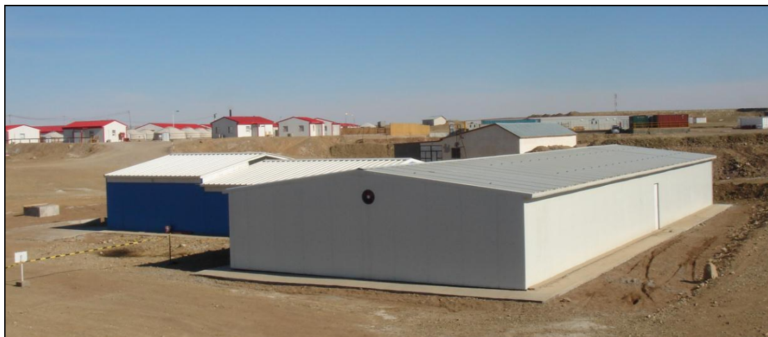
Figure 4.20: Completed Wastewater Treatment Plant (including expansion)
