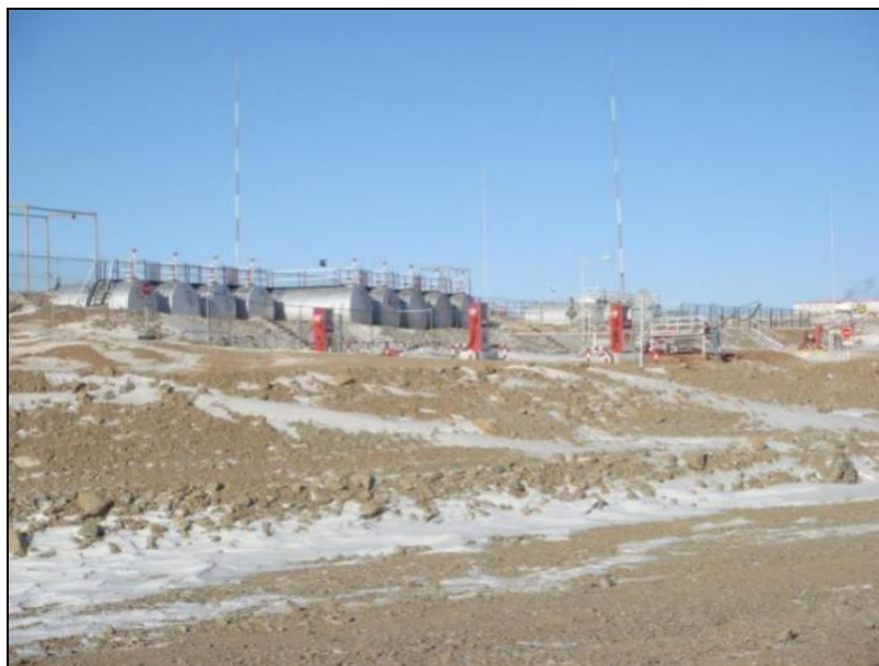
Figure 4.23: Current Petrovis LLC Bulk Fuel Store
