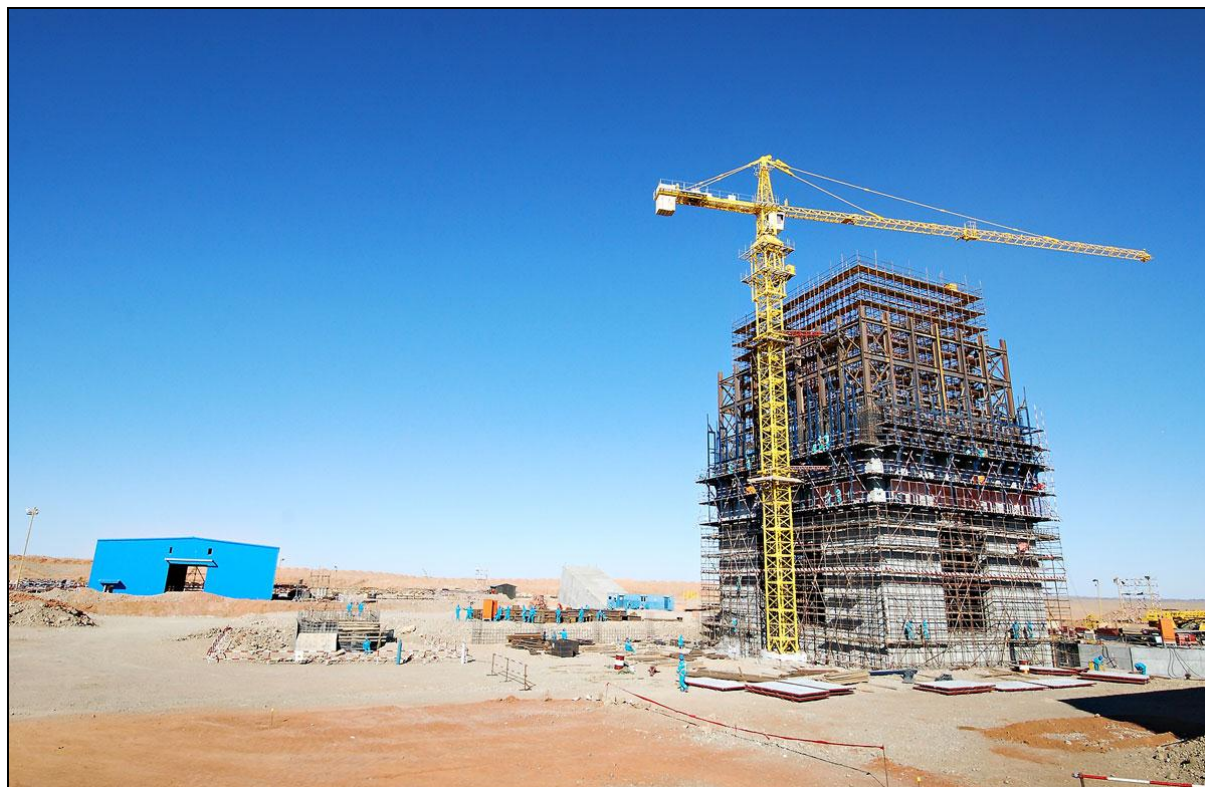
Figure 4.3: Shaft 2 in Construction, March 2011
