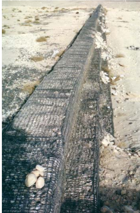
Figure 4-9: Structure of retardation dyke, composed of stone-contained gabions
