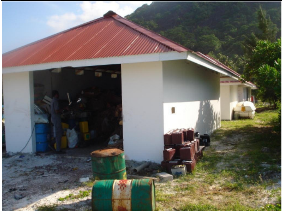
Photo 1 Solid Waste Store near the harbour
