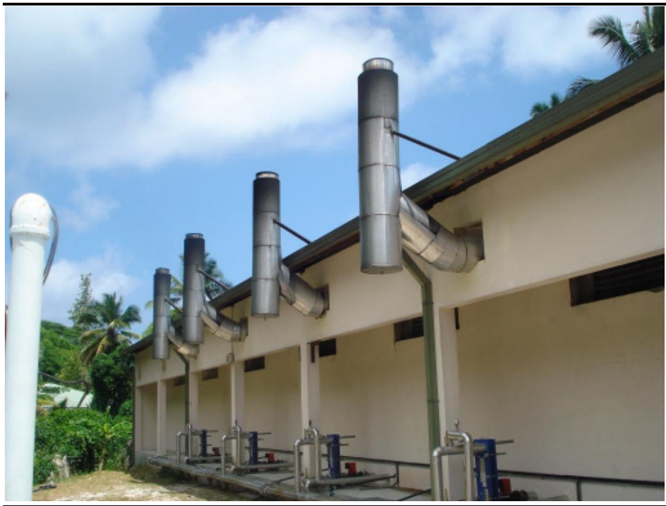
Photo 6 Generator Exhausts
