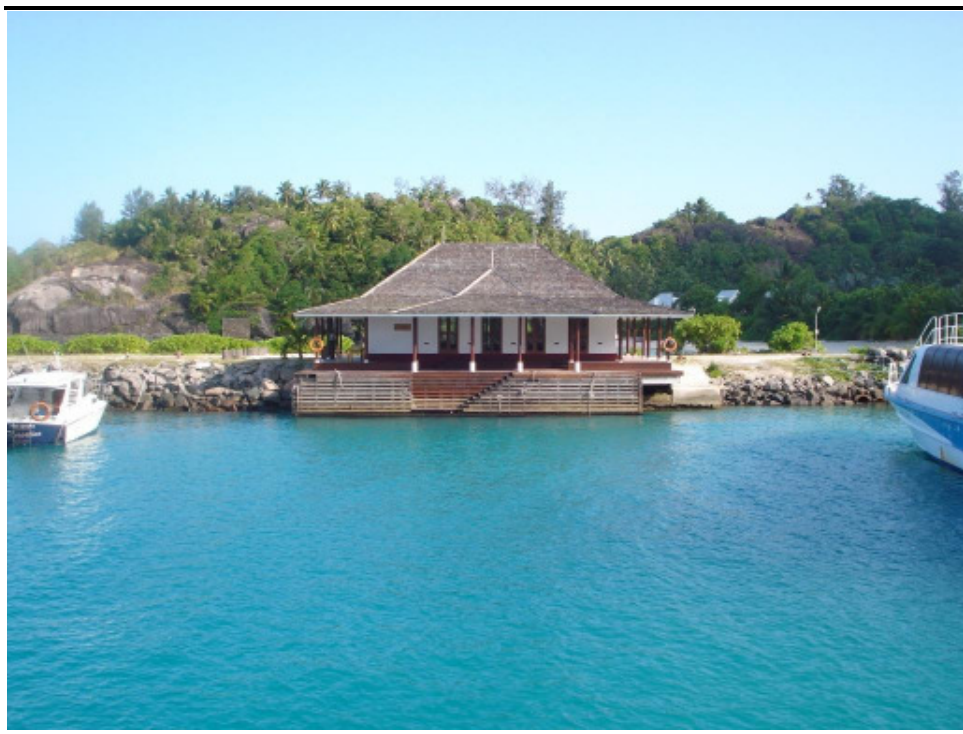
Photo 4 Resort Welcome Jetty Facility
