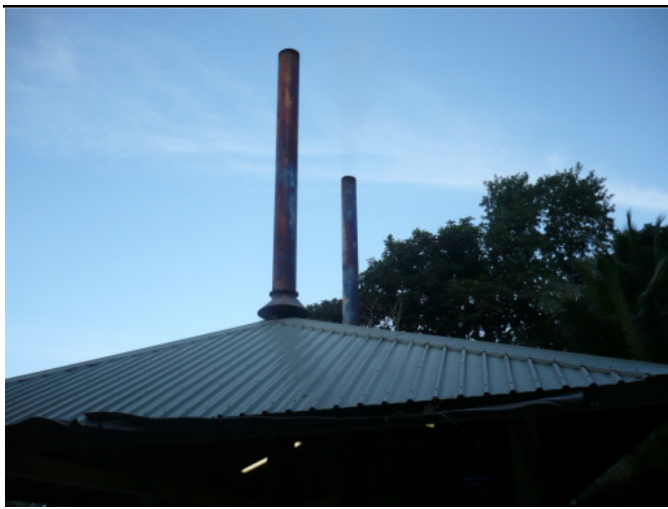
Photo 24 Incinerator chimney stacks
