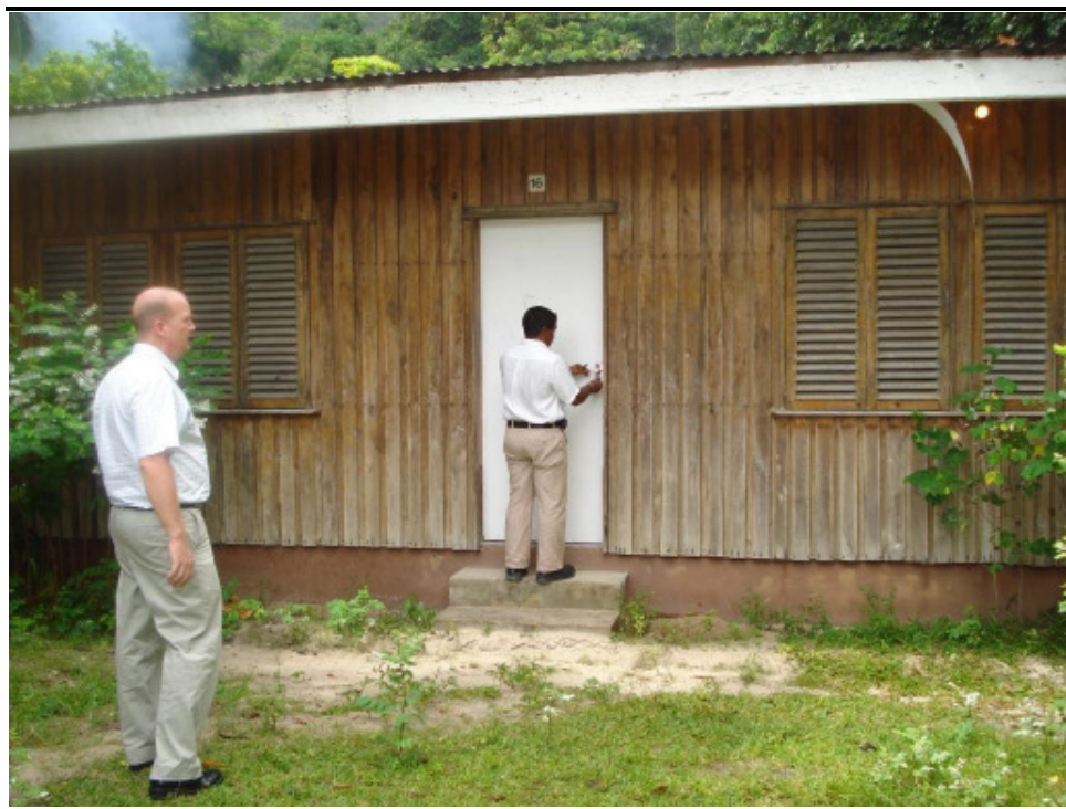
Photo 10 Offsite Chemical Store
