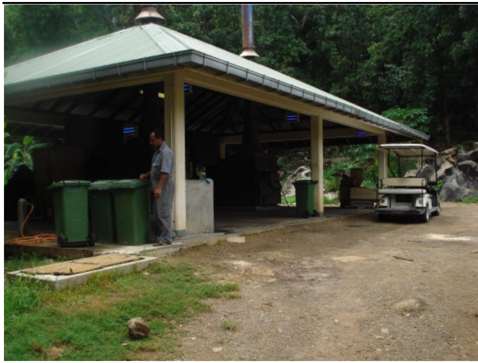
Photo 14 Solid Waste Handling Area and Incinerator units
