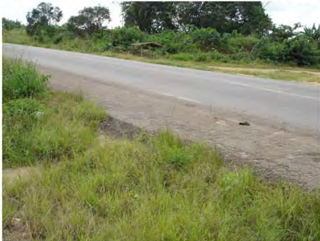
Photo 5.5.1 RN3 condition outside project site
