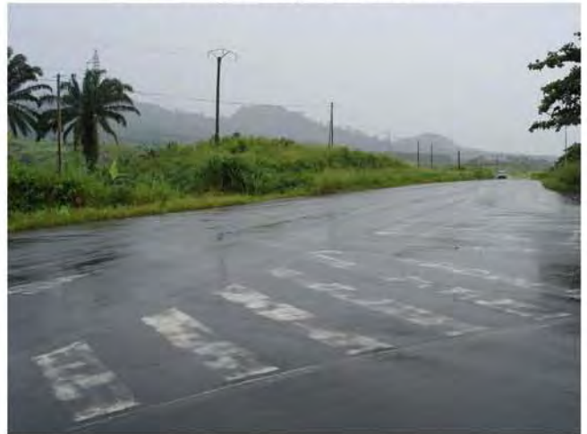
Photo 5.5.16 Access to AES Sonel's powerplant at Limbe
