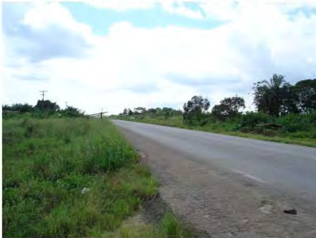
Photo 5.5.3 Site access visibility (left)
