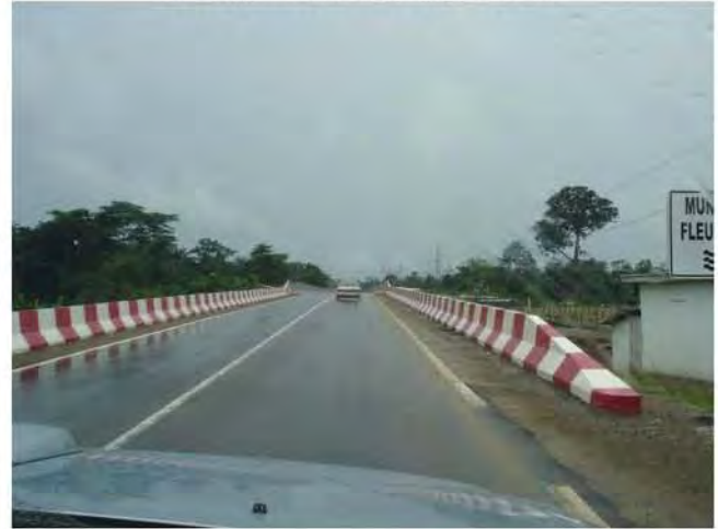
Photo 5.5.14 Westbound on Bridge over Mungo River
