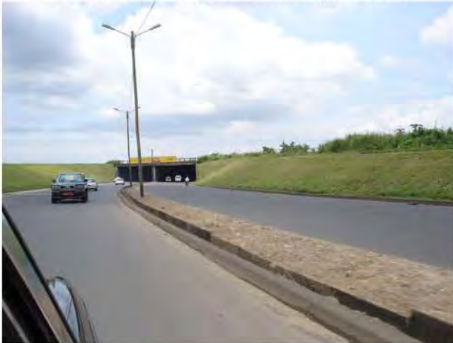
Photo 5.5.9 Airport Runway Overpass along RN3 exiting Douala
