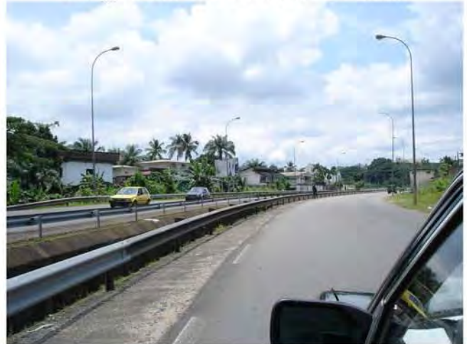
Photo 5.5.10 Dual-carriageway along Boulevard Beseke in Douala
