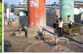
Venkatapur – Water Supply – For Drinking/General Use
