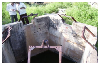
Jettur – Govt. Well – For Drinking/General Use
