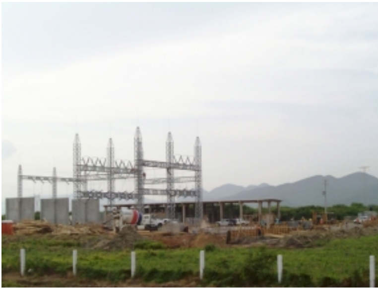
Photo of the substation footprint
