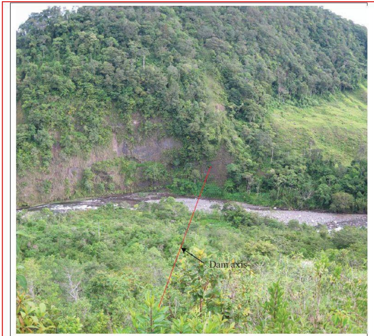
Photo 5: Monte Lirio dam site.
