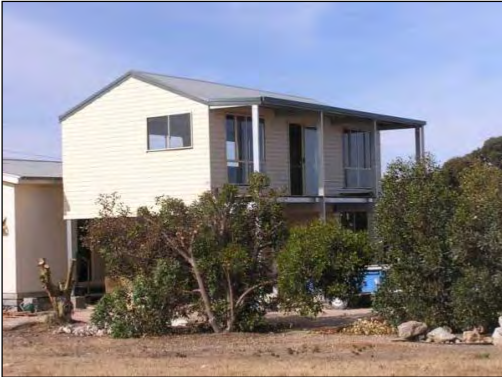
Figure 13.6 – Example of the steel-framed housing being considered by the Relocation Task Force.
