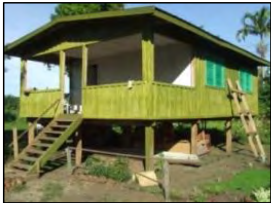
Figure 13.48 – Pitukoli Primary School
