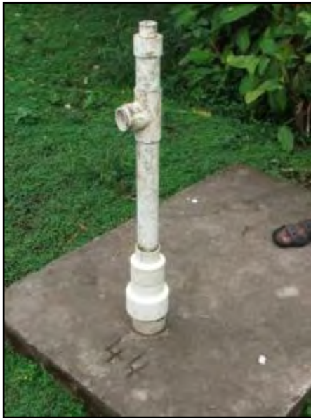
Figure 13.37 – Village boreholes provided by GRML.
