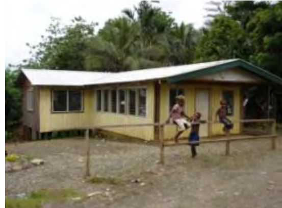
Figure 13.11 – Upgraded Community Centre at Obo Obo.
