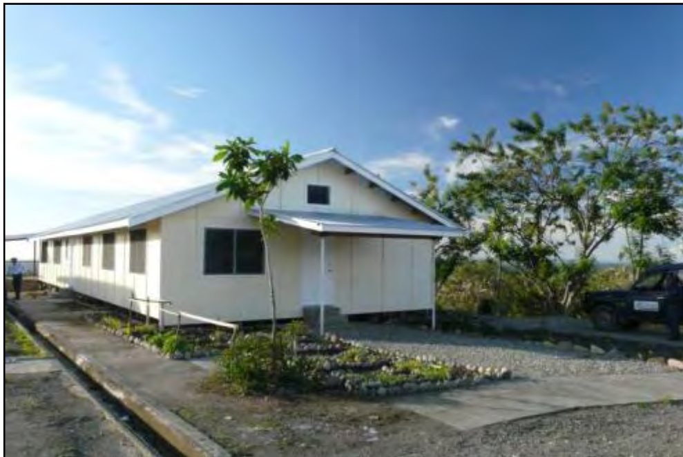
Figure 13.7 – Newly constructed Community Relations Department building providing easy access for the community.
