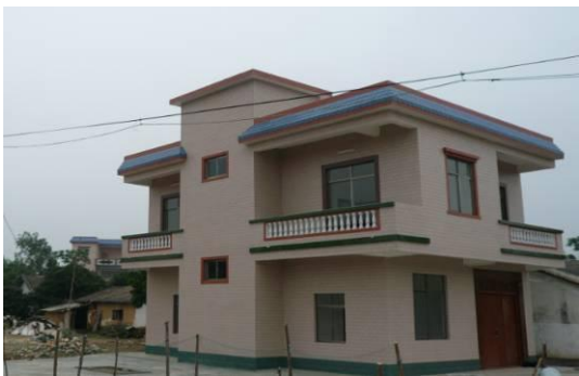
Picture 17 New Building (2010)
