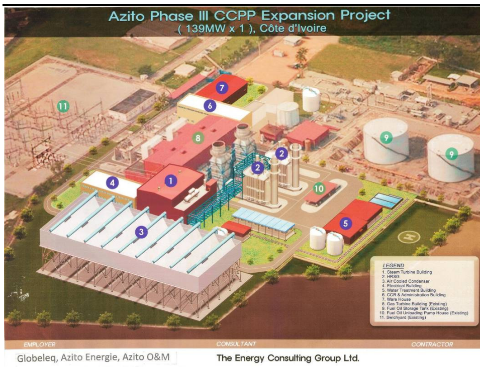
Figure 2.5 Overall project concept including phase III expansion
