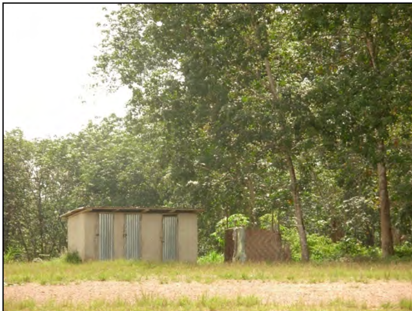
Figure 7-25: Toilet and bathing facilities within Camp 5.
