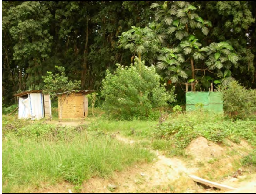
Figure 7-15: Toilet and bathing facilities within Camp 2.
