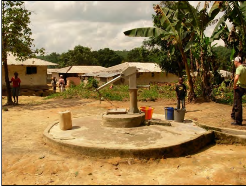
Figure 7-19: A well in Camp 3 with cement cover.
