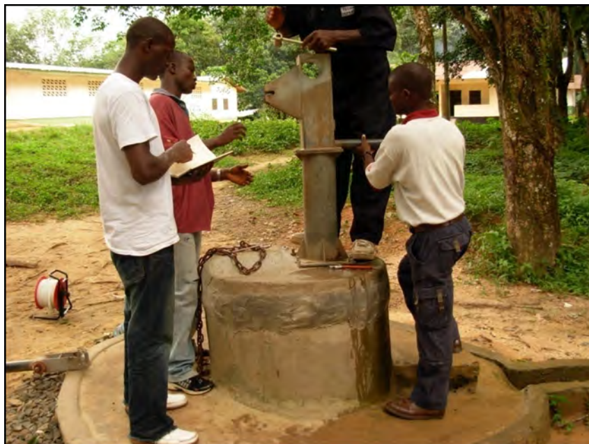
Figure 7-26: Well with cement cover in Camp 5.
