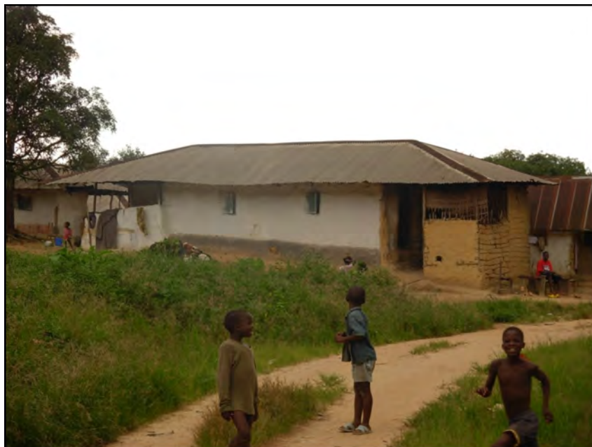
Figure 7-18: Note the added section to the house that is made of mud and sticks. This section serves as a kitchen for the household residents.
