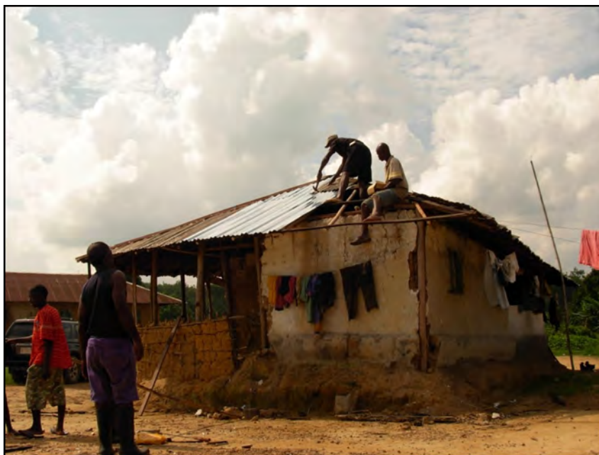
Figure 7-13: Basic renovation for one of the houses in Camp 2.
