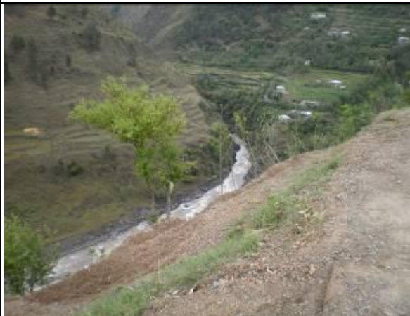
Downstream Flow of Kunhar River near Boi Village Showing Deeper Bed and high Banks of the River - 2010
