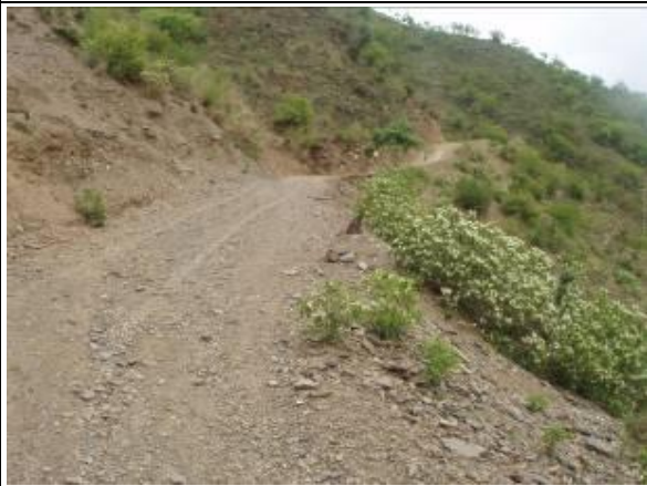
A katcha Track where Maintenance Road is to be Constructed - 2010
