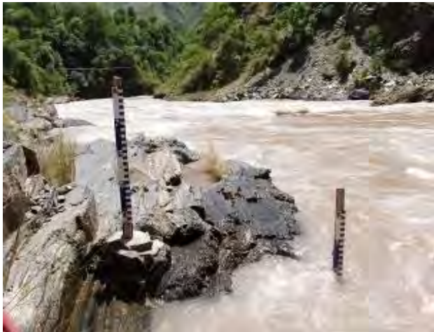
Gauge Installed at Weir site - 2006
