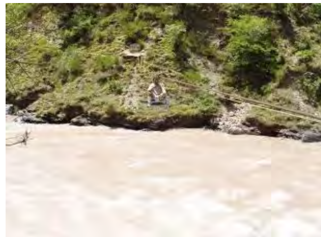
Cable way on Kunhar River at weir site - 2006
