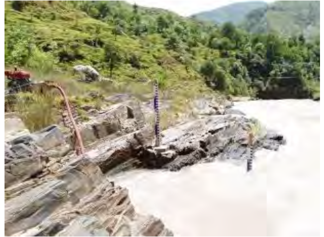
Gauge Installed at Weir site - 2006
