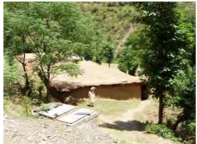
House to be Affected due to Diversion Tunnel at Weir Site -2010
