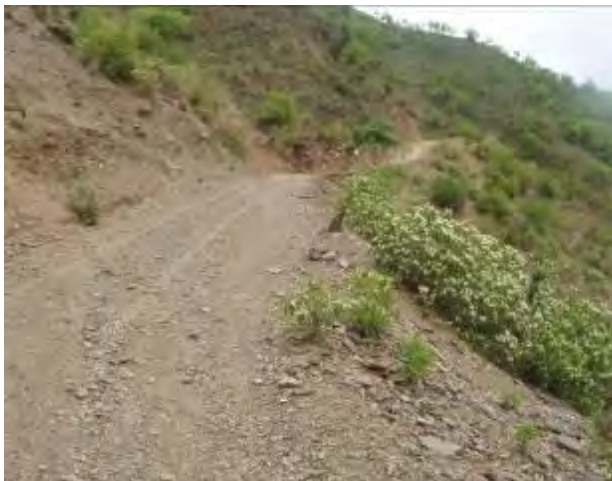
A katcha Track where Maintenance Road is to be Constructed - 2010
