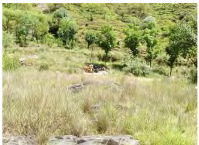
Drilling process at Weir site - 2006
