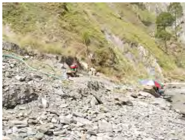
Drilling in process at Powerhouse site - 2006
