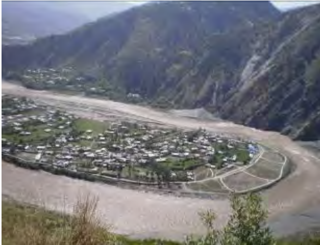
View of Powerhouse Site - 2010
