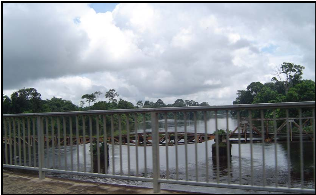
Bridge over the Nyong River
