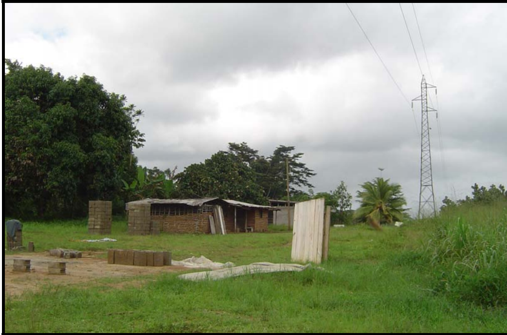
Existing Power Line at Mpolongwe
