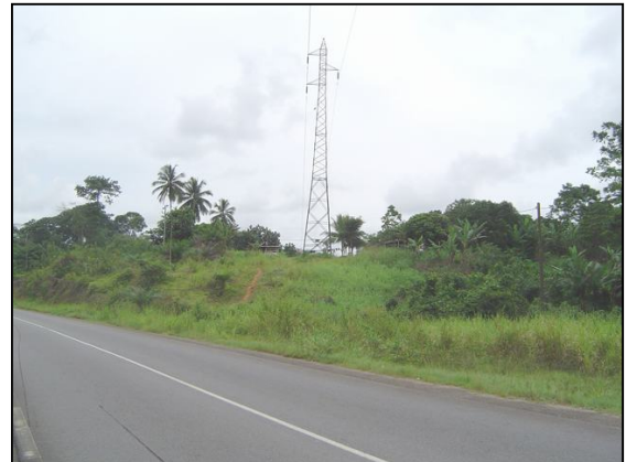
Photo 5.11.4: 90kv pylon and wayleave at plant site
