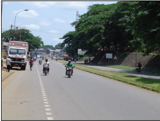
Photo 5.7.4: Road through Edéa
