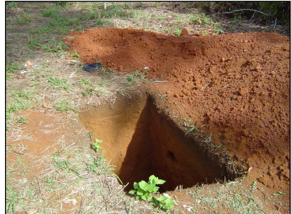
Photo 5.8.1 Trial pit on plant site
