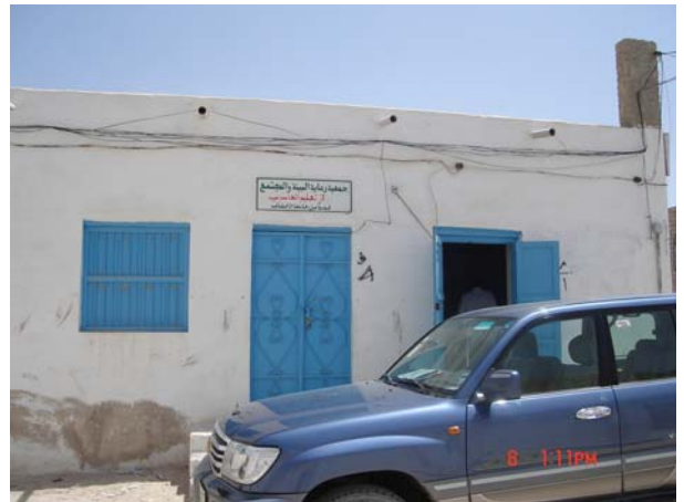
Figure ( 28 ) Show Building of Environment and Social protection Society-Al-Naqa'a
