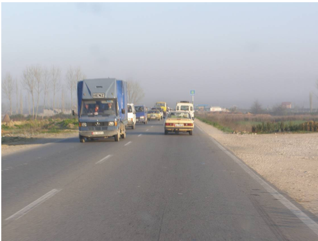
Figure 27 Traffic on Road Vore - Fushe Kruje
