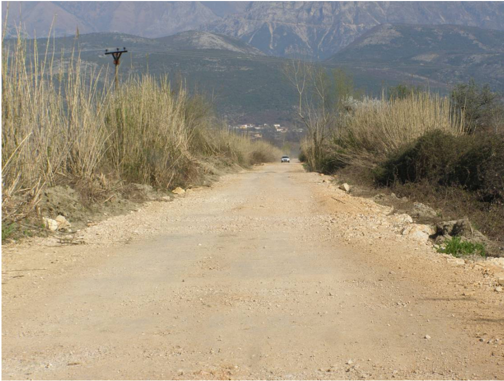
Figure 37 Burizane Access Road – Unpaved Section
