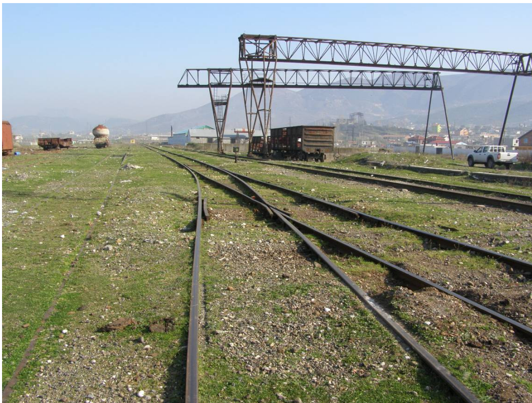
Figure 23 Gjorm Yard - Turnout
