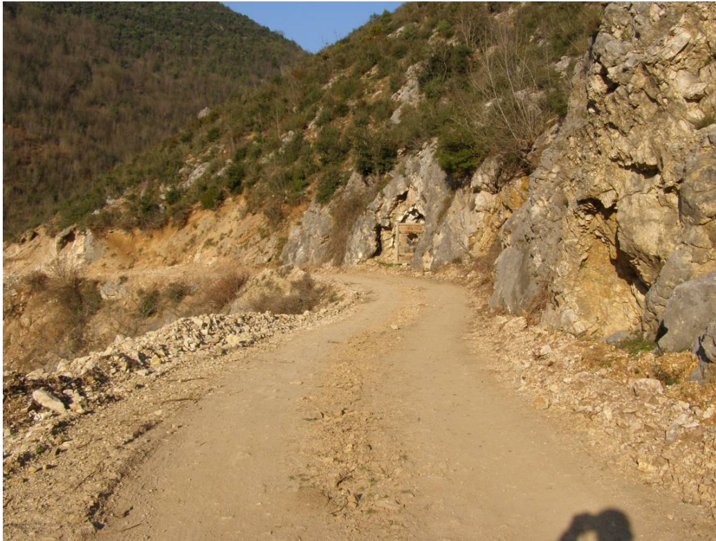
Figure 41 Road Mamuras – Cement Plant / River Drojes Bridge Location
