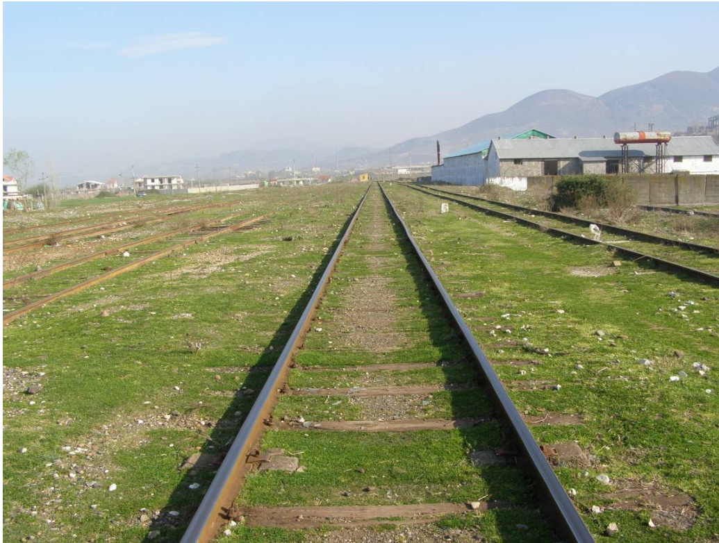
Figure 22 Gjorm Yard – Northern Access
