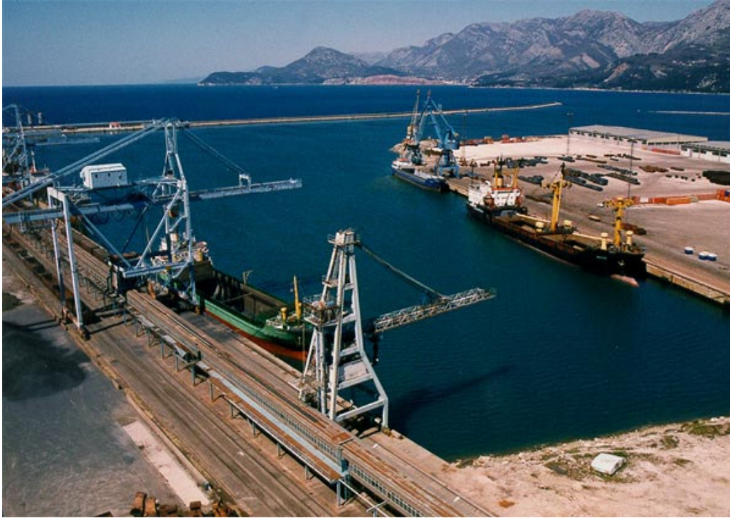
Figure 16 Bar Port – Loading Facilities
