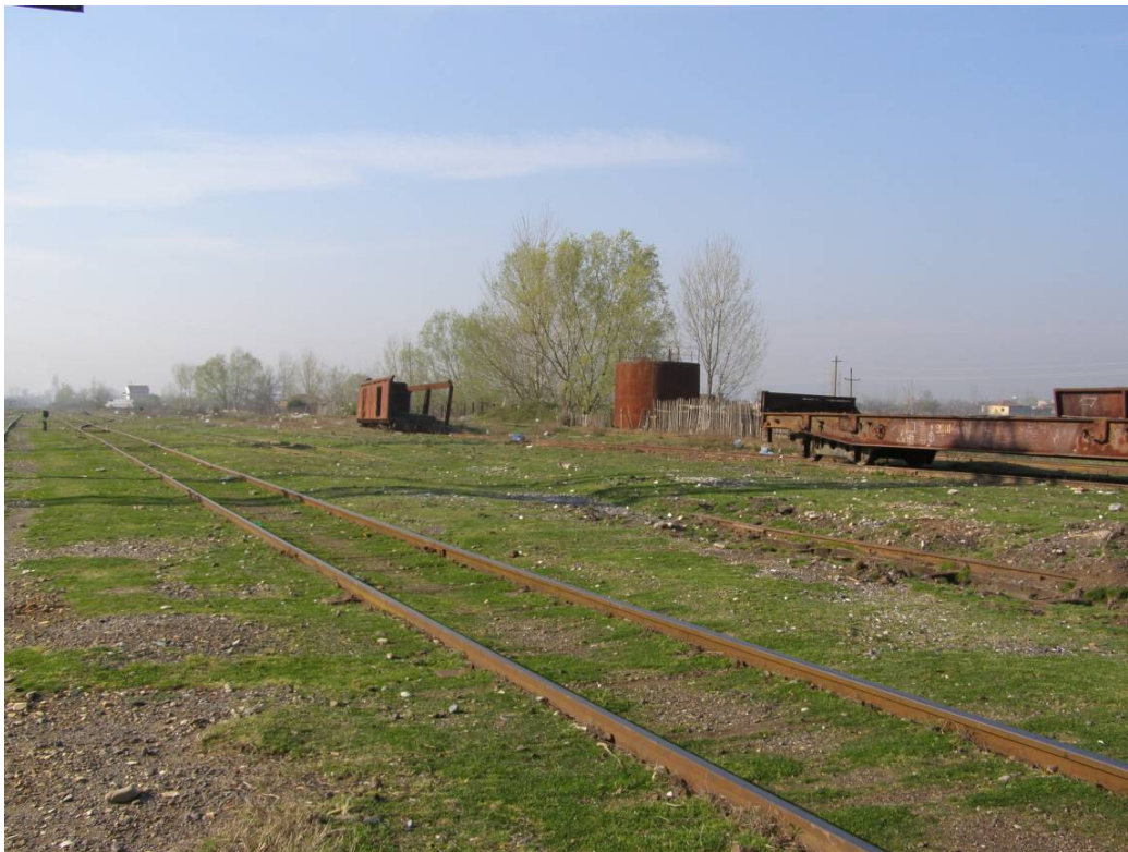
Figure 21 Gjorm Yard – Rail Sidings
