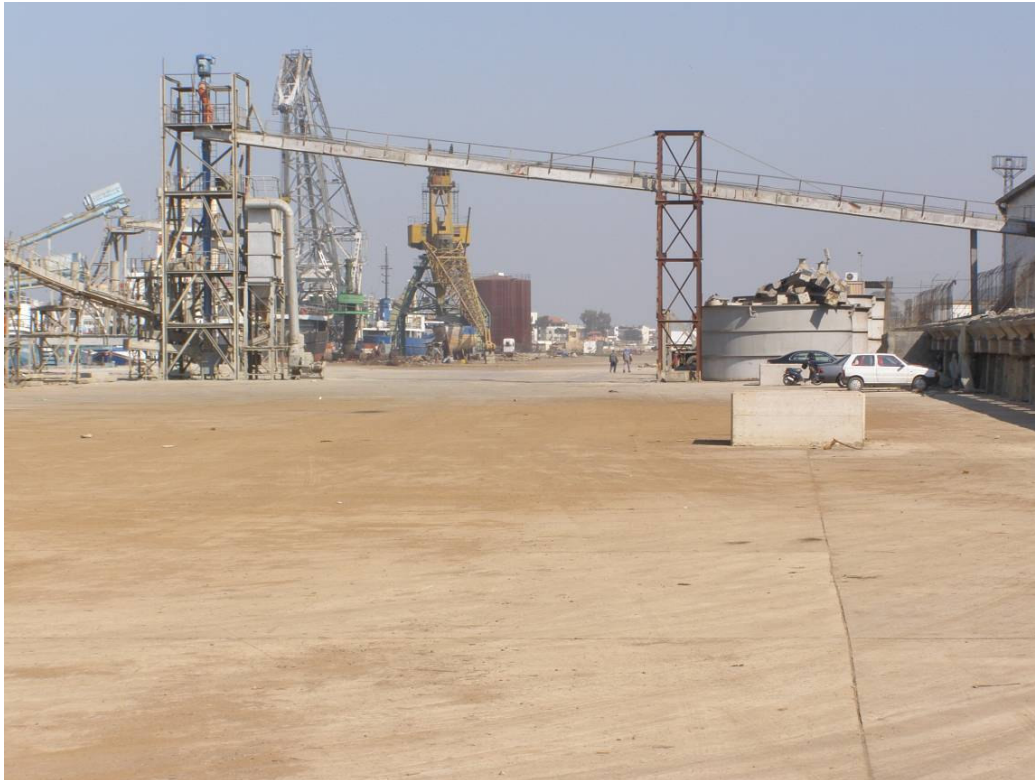
Figure 10 Durres Port – Eastern Pier – Loading Facilities
