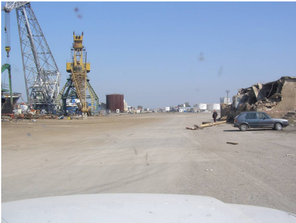
Figure 7 Durres Port – Eastern Pier – General View
