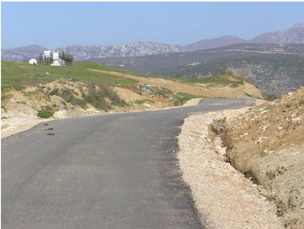
Figure 38 Burizane Access Road – Paved Section
