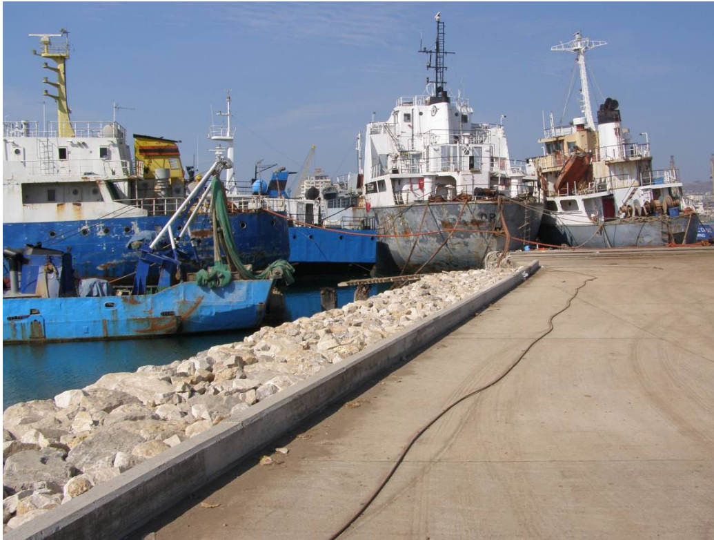
Figure 8 Durres Port – Eastern Pier – Southern Dock
