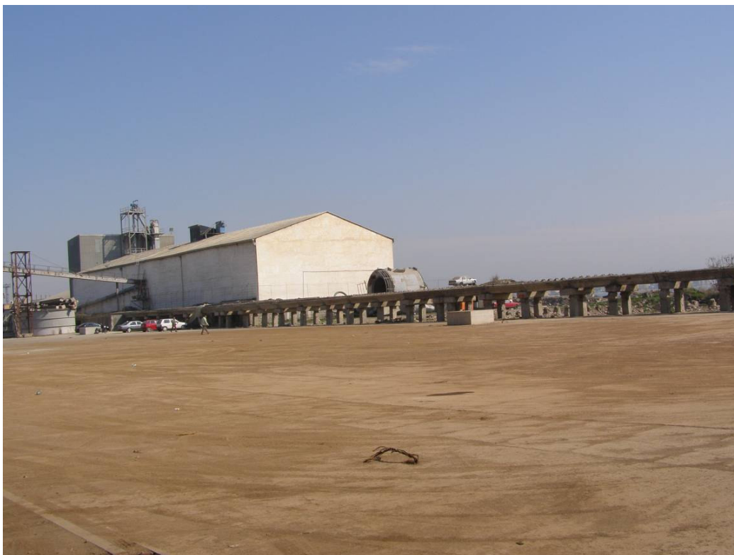
Figure 13 Durres Port – Eastern Pier – Abandoned Elevated Rail line
