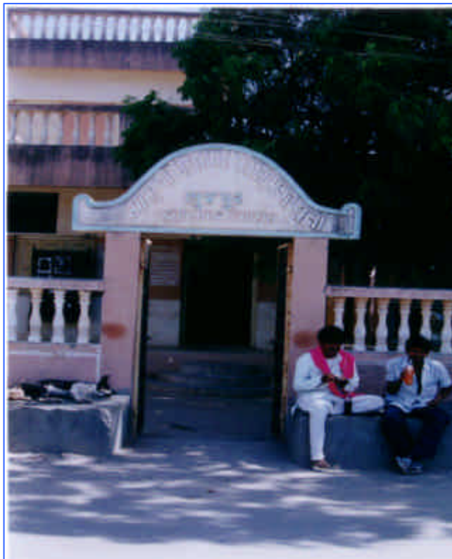
Figure No.3 Gram Panchayat Office, Bhojpar
