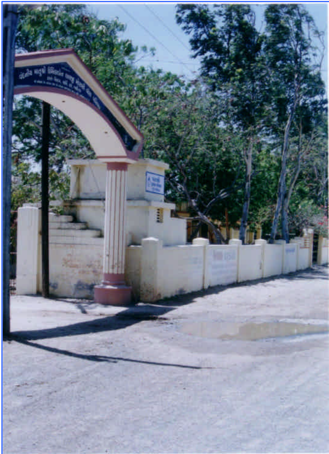
Figure No.9 Primary School at Navinal
