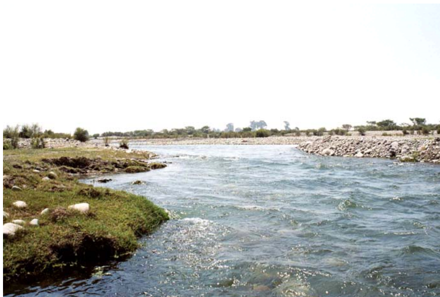
Figure 2. View of Pisco River KP 334+800
