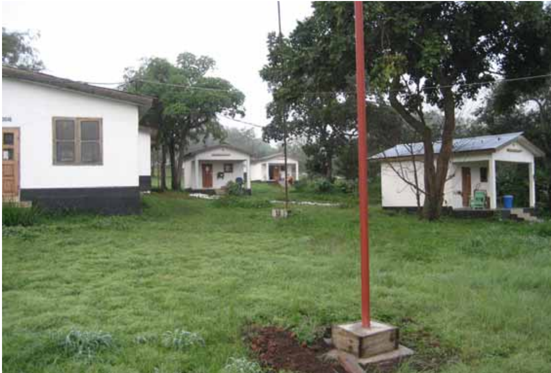
Photo 7 Existing Infrastructure at the Canga East Camp
