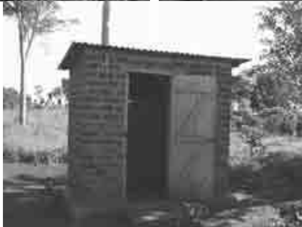
A Ventilated Improved Pit (VIP) two-stance latrine is provided
