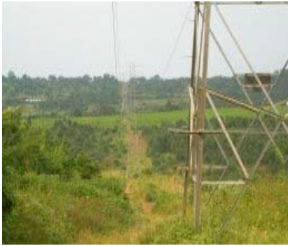
a) Pylon 51 facing towards the tea plantations
