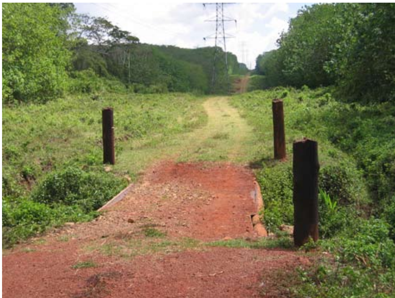
Recently-upgraded bridge over the Waliga River between Towers 169 and 170 (January 2006)
