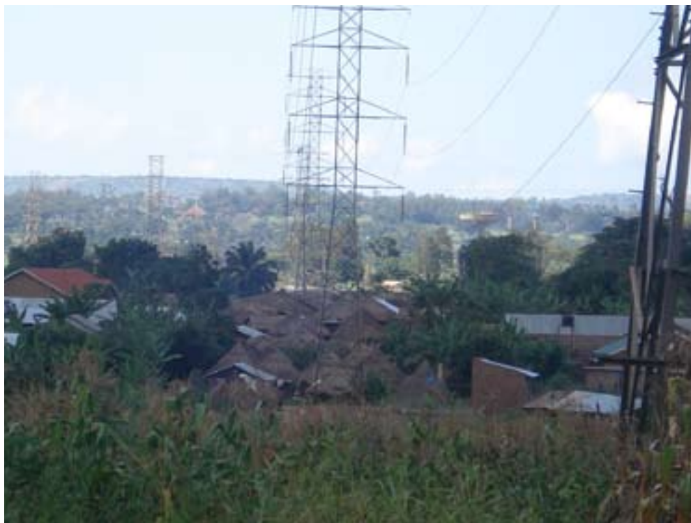
Example of dense land use in vicinity of Nalubaale Substation.
