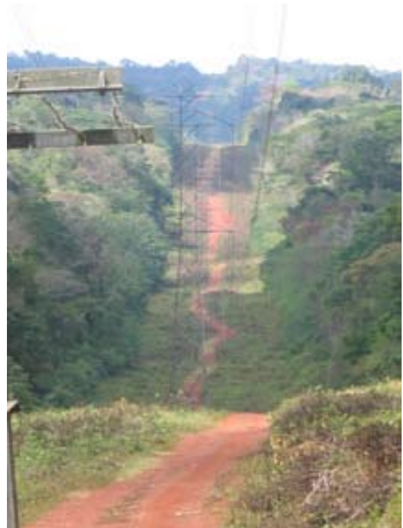
Tower 154 west looking towards Tower 153 (January 2006)
