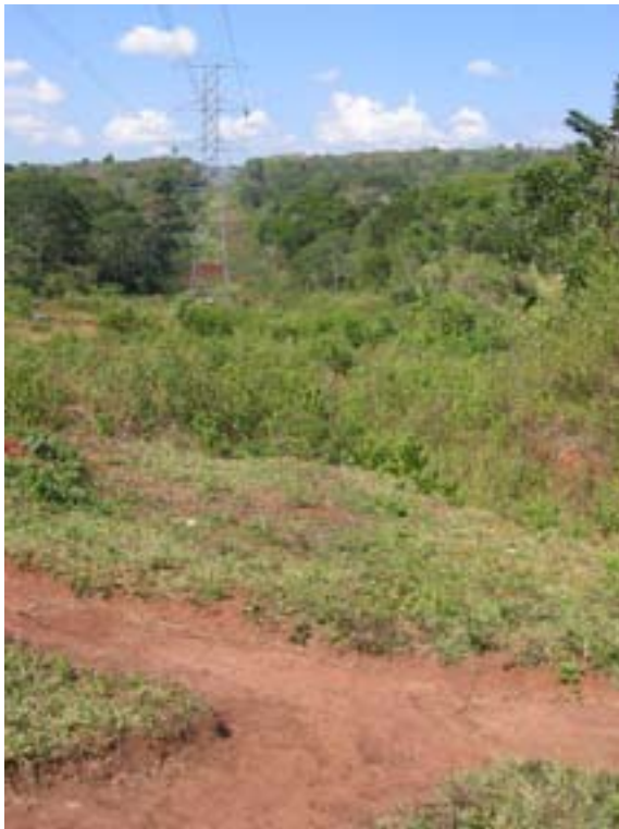
Tower 138 Ssese looking west (January 2006)
