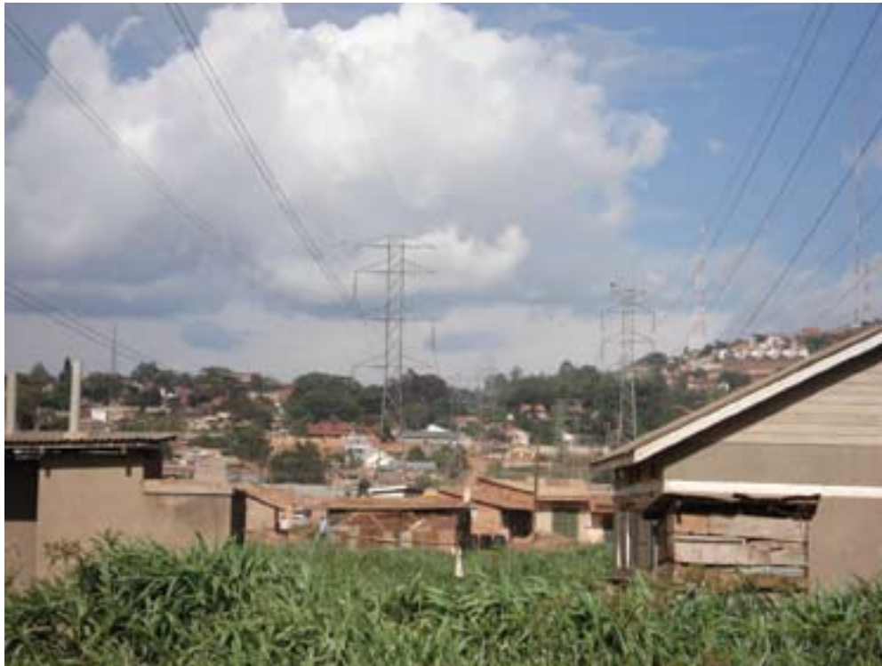
View of 132kV corridor in vicinity of Kampala North Substation.
