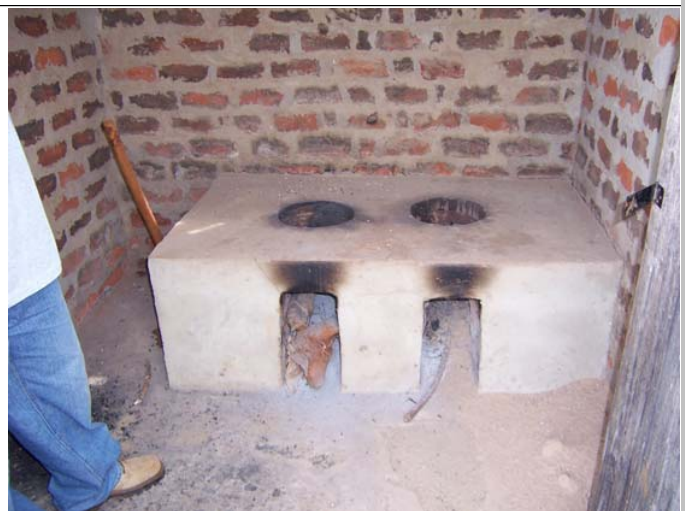
Pilot improved stove installed by AESNP to rationalize firewood use – January 2006
