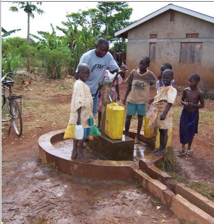
Site water well with operational Orbit hand pump – January 2006
