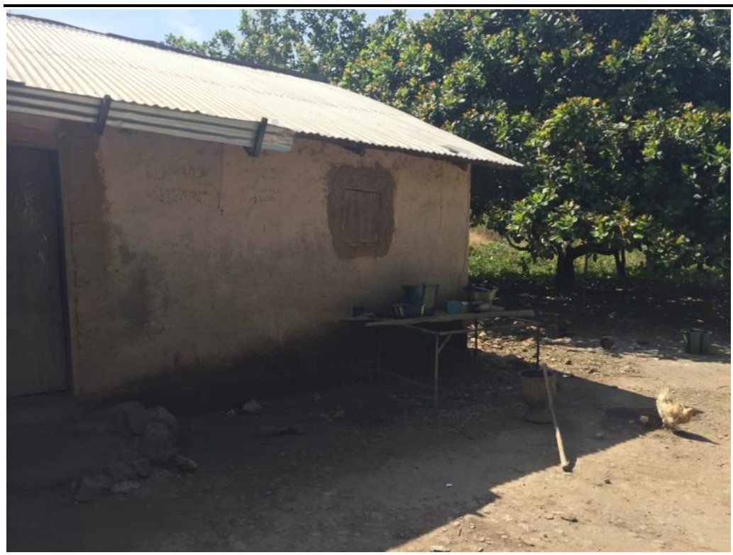
Figure 3.36 House located within the water pipeline route (PL22)
