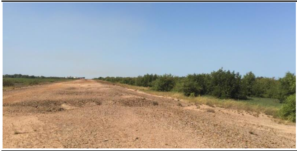
Figure 3.75 General view of the cleared area in the coastal section of the GAC platform
