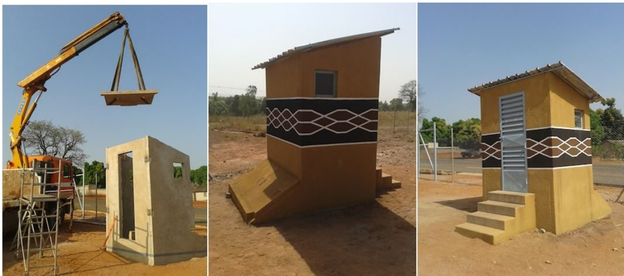
Figure 18 – Design Example – Double Pit VIP Latrine
