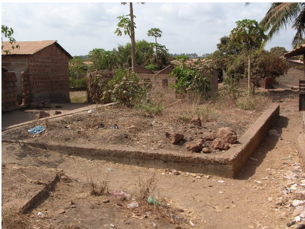
Foundation: two to three rows of bricks are placed to materialise someone's "ownership" of a land plot
