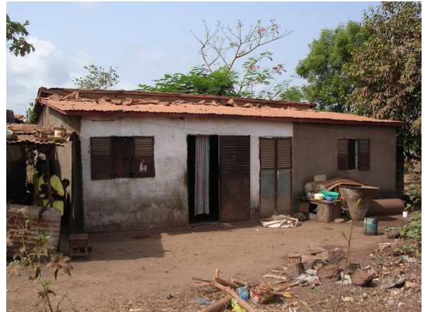
Typical Dapraass house (the left apartment is used by the owner, while the right side, added later, is dedicated to rental)
