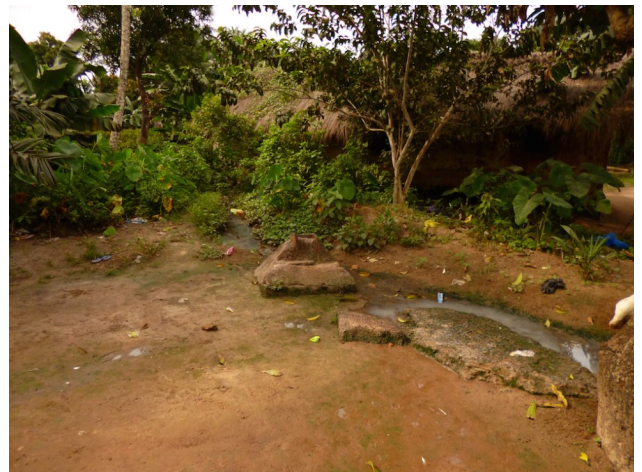
Poor drainage of waste and grey water can potentially result in health issues, including cholera and other water borne diseases
