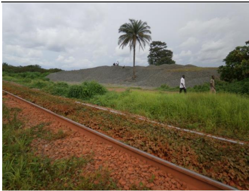
Figure 1.10 Pile of gravel on rail's edge, Madina Carrefour
