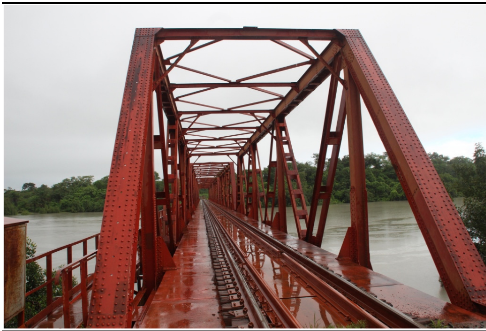
Figure 4.12 Bridge over Rio Nuñez River (just after KP44)
