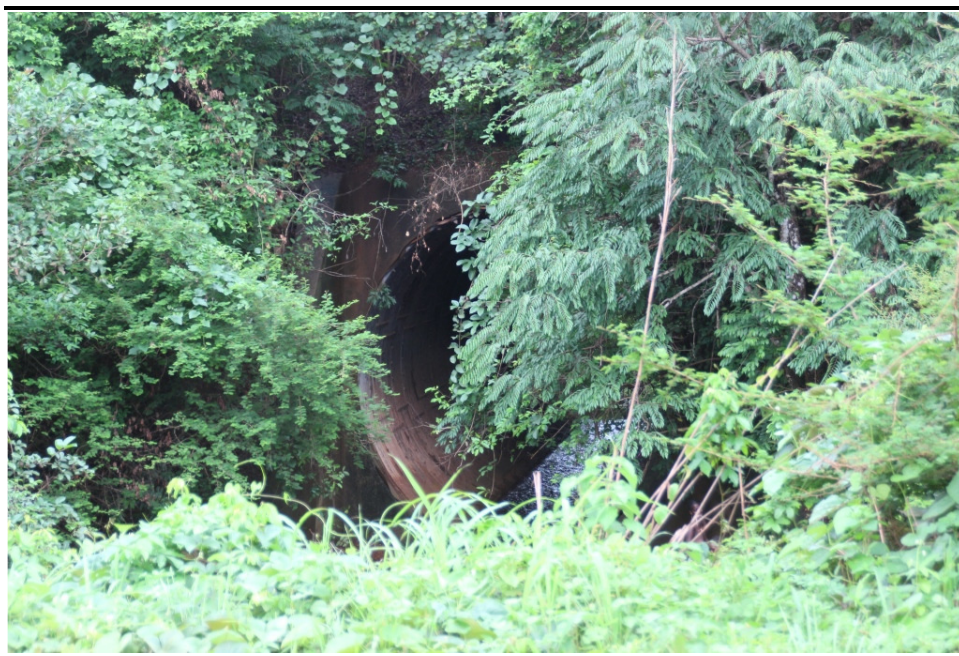
Figure 4.16 Culvert at KP77
