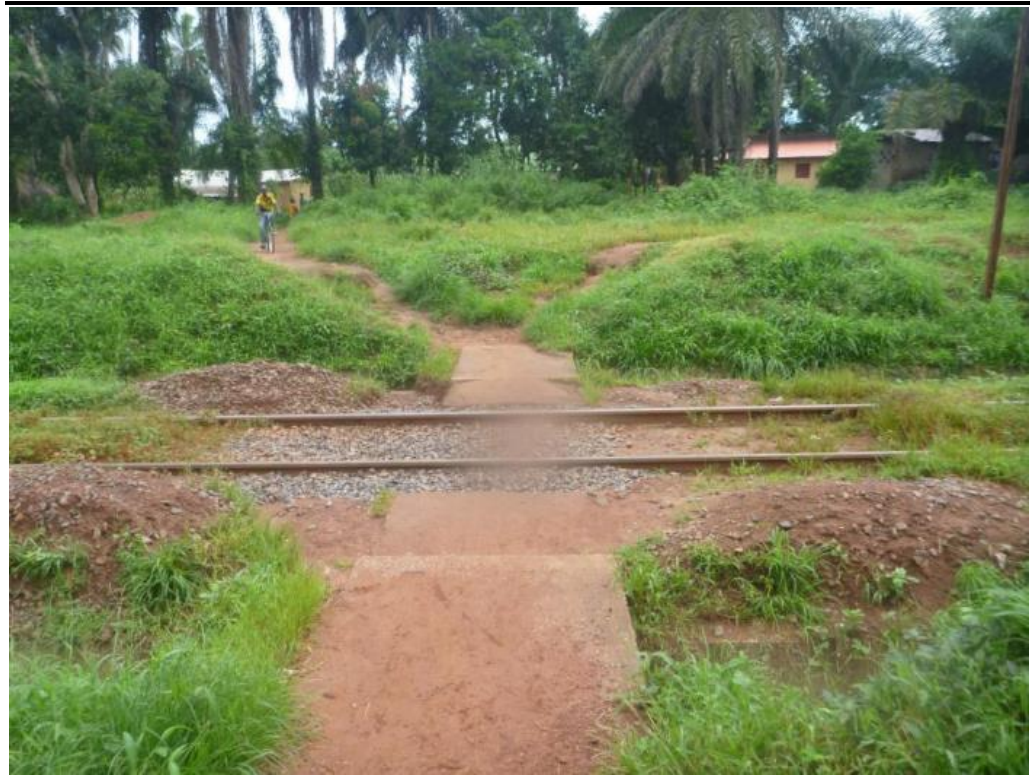
Figure 1.5 Crossing for pedestrians and two-wheelers, Kolaboui
