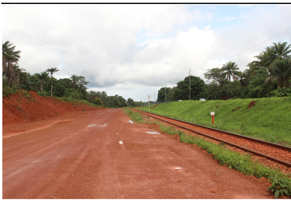
Figure 2.4 Excavation work at KP 27
