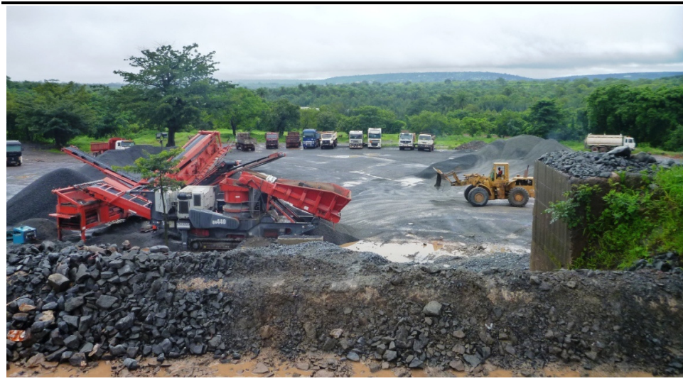
Figure 4.22 Quarry material crushing area at Dabis-Kasongony quarry, Dabaya
