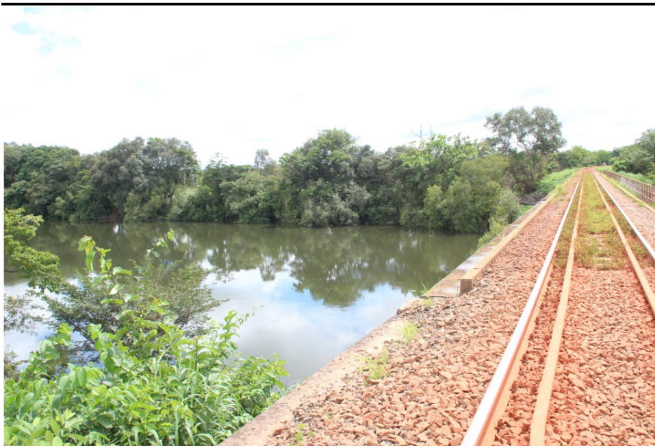
Figure 4.6 The Tinguilinta River crossed by the railway at around KP78
