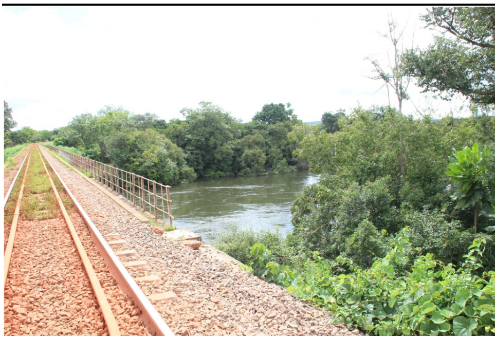
Figure 4.13 First bridge over the Tinguilinta River (KP78.5)
