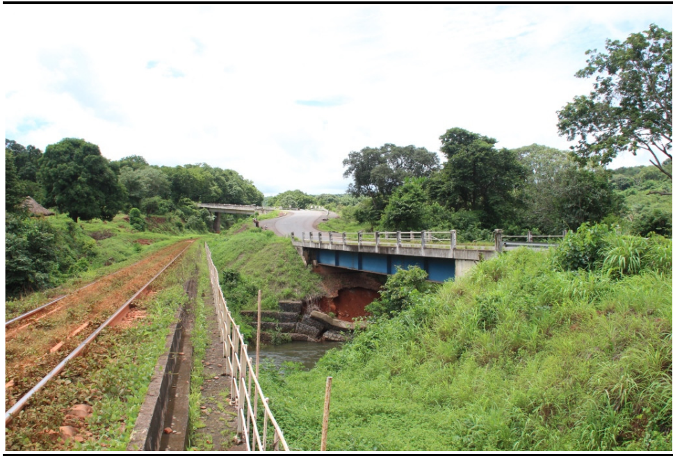
Figure 4.14 Bridge over the Kéwéwol River (around KP106.5)
