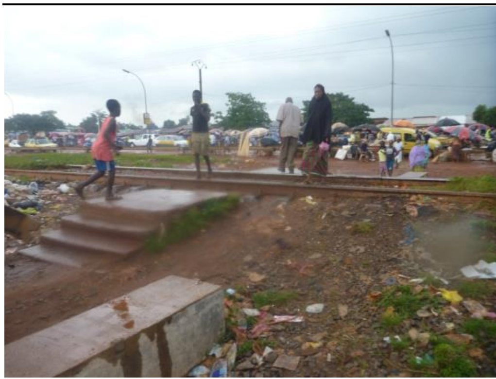
Figure.1.2 Pedestrian crossing at the level of the Sahara market and foundation of the future pedestrian bridge
