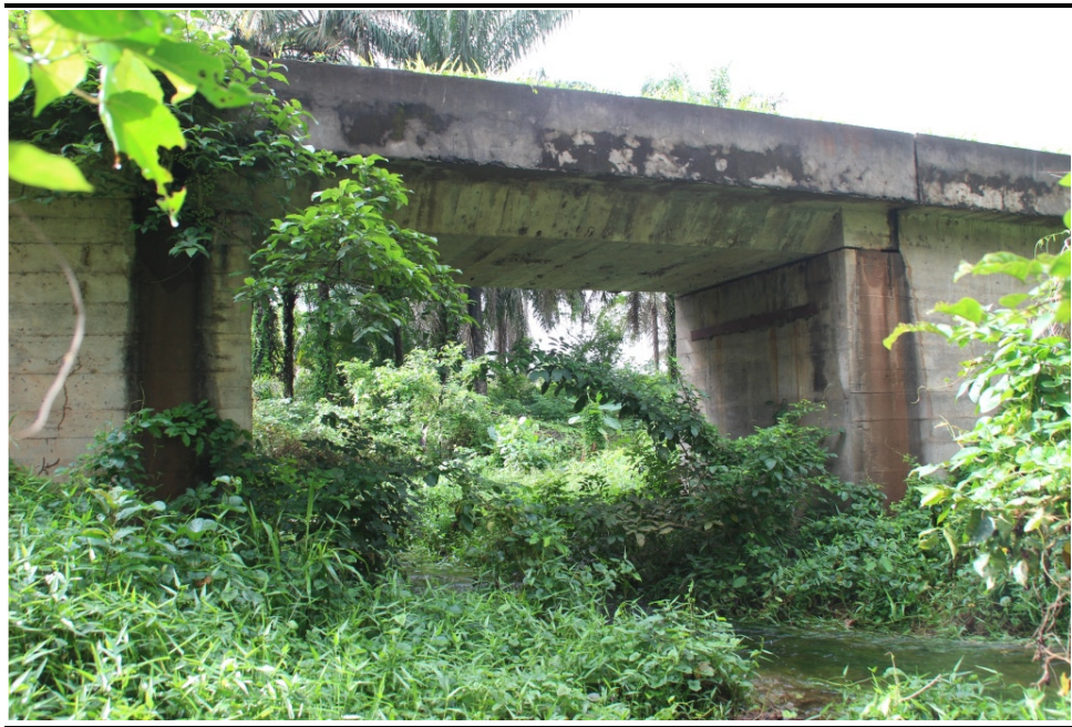
Figure 4.15 Bridge over a small water course at KP36.4
