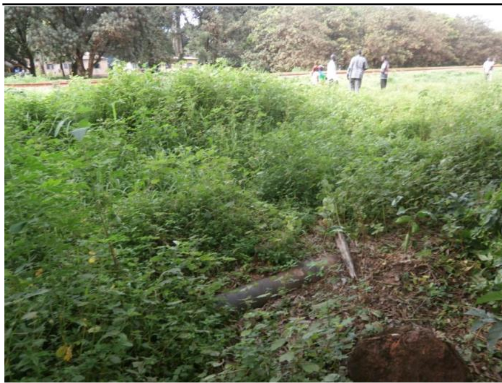
Figure 1.9 Water pipe at level of railway, Madina Carrefour
