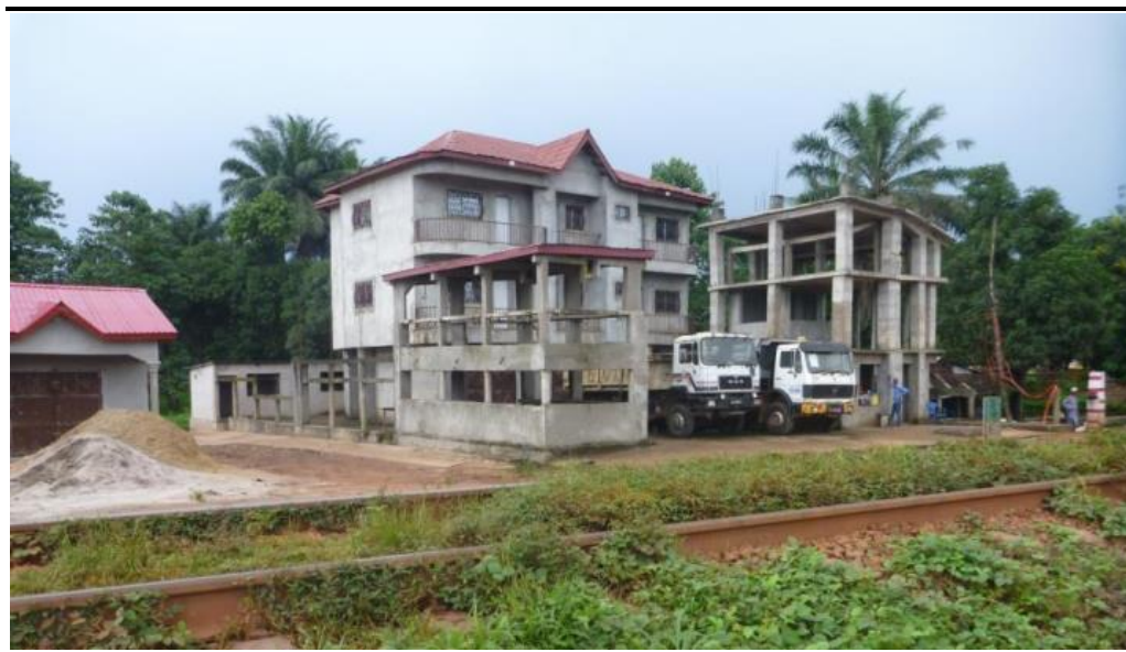
Figure 1.6 Two-storey building in the 50 m corridor, Kolaboui
