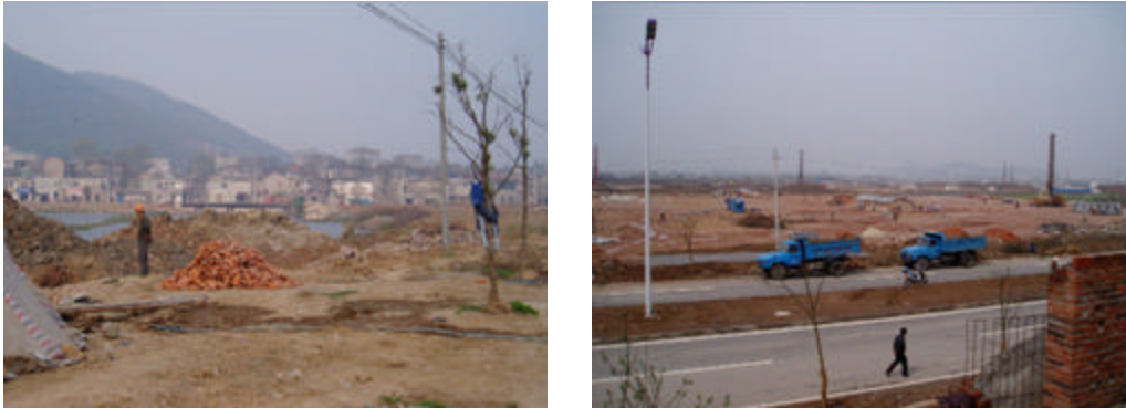
Figure5-1 The replacement site is currently under construction
