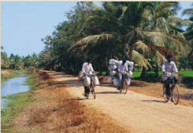
Bypass road near Ravva plant
