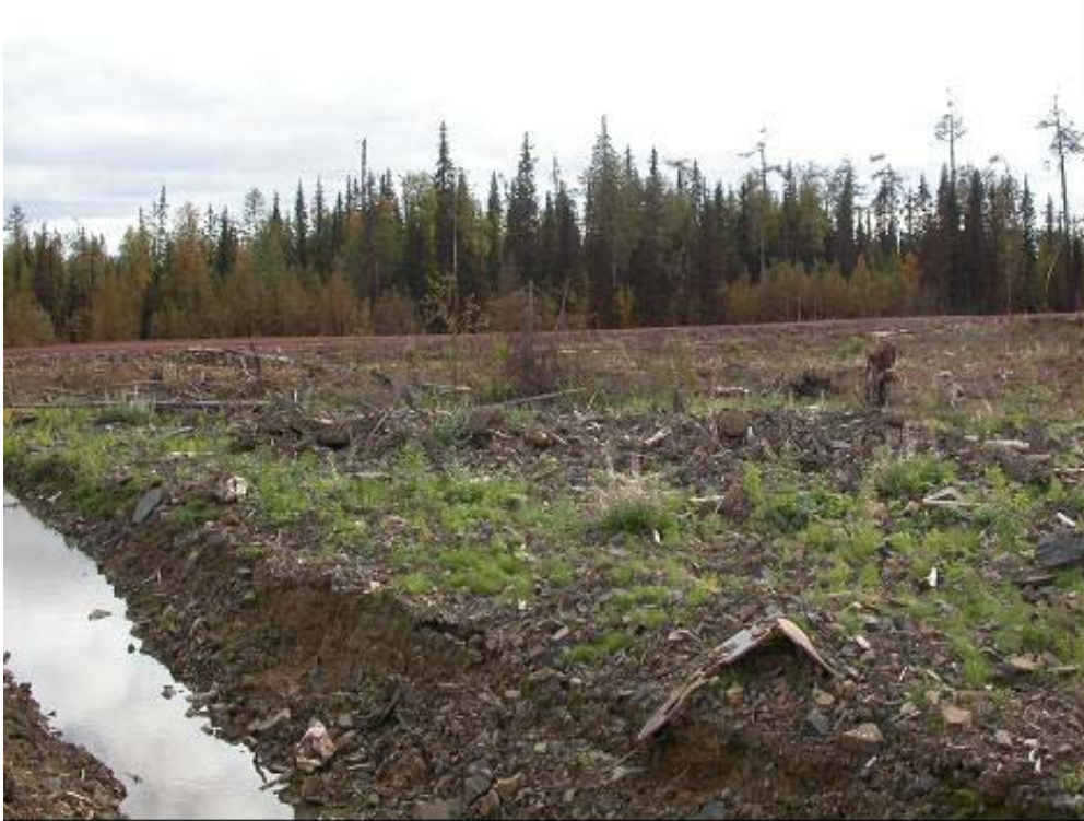
Plate 8: Clearing of forest for the purpose of pit excavation, showing the effects of unconsolidated soils and concomitant erosion risk
