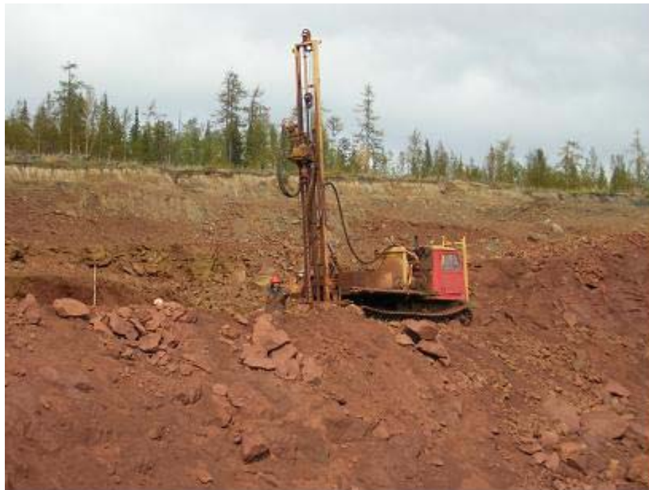
Plate 1: Drilling operations to characterize the areas to be mined
