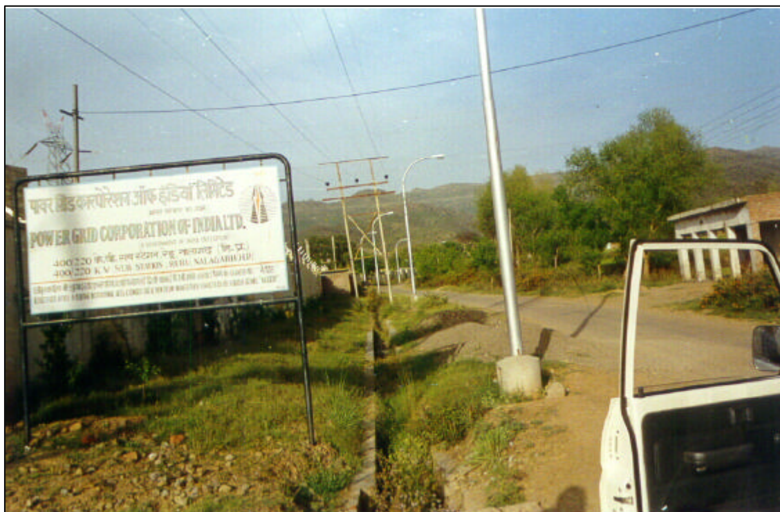
Nalagarh Power Station where the proposed Transmission Line will feed the National Grid from ADHEP
