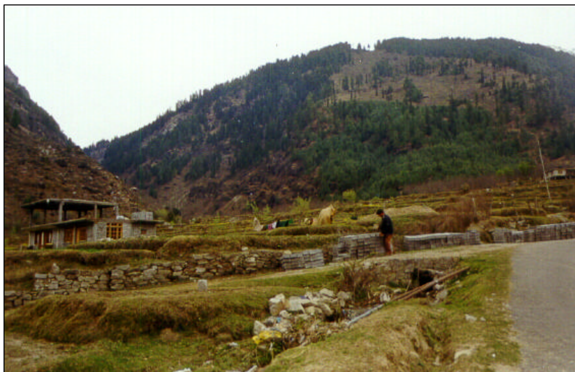
View of the area near the switchyard at the transmission line starting point
