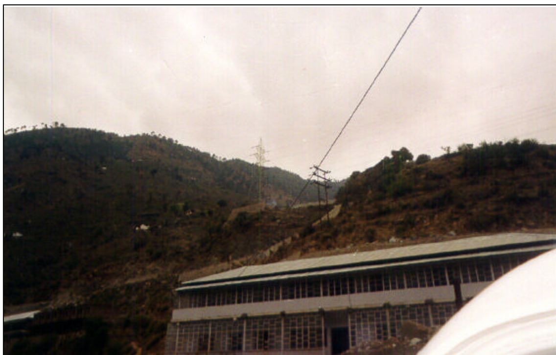
Location near Pandoh village where the proposed line would cross NH-21
