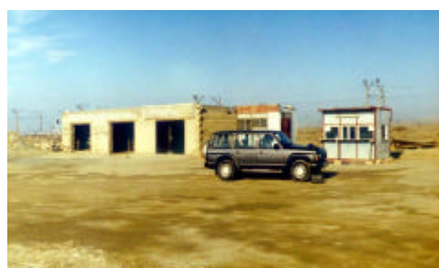
a) Garage structure & moveable stalls
